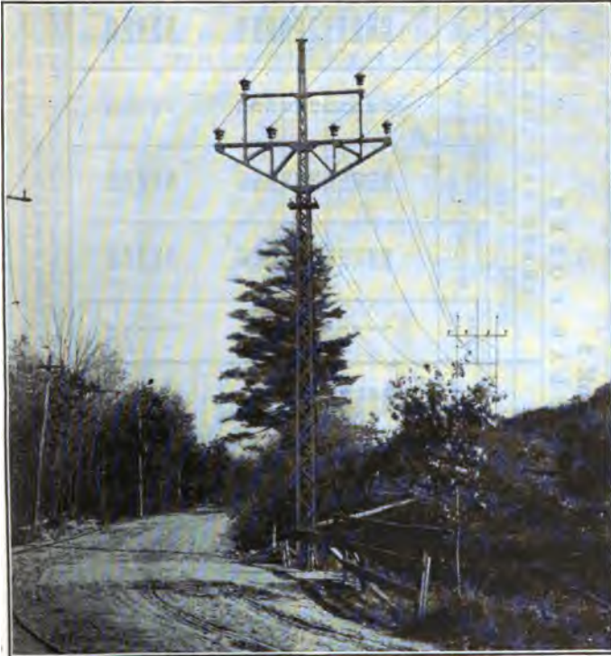
FIG. 44.—Double circuit three-phase 66,000 volt steel pole.
