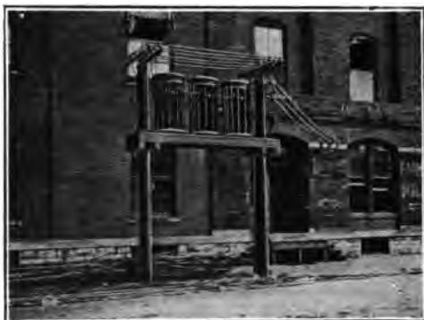
FIG. 406.—Special transformer rack.
