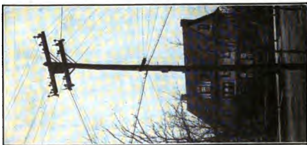
FIG. 414.—Consumers' service open wire and duplex cable.
