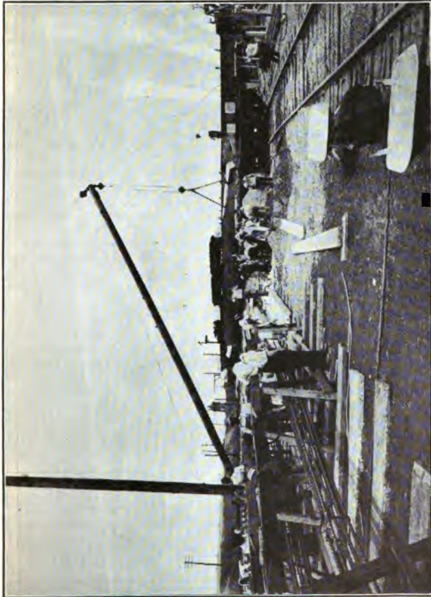
FIG. 34.—Forms for concrete poles and method of loading for transportation.
