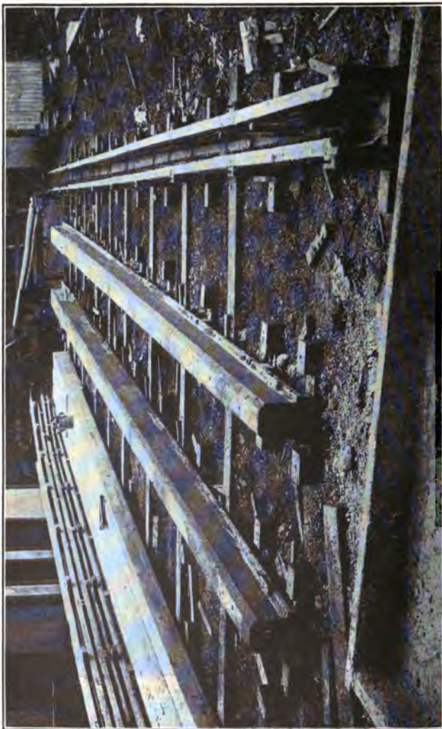
FIG. 35.—Solid concrete pole forms (Illustrates various stages of manufacture.)
