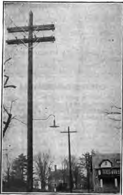
FIG. 420.—Single wire incandescent lamp leads.
