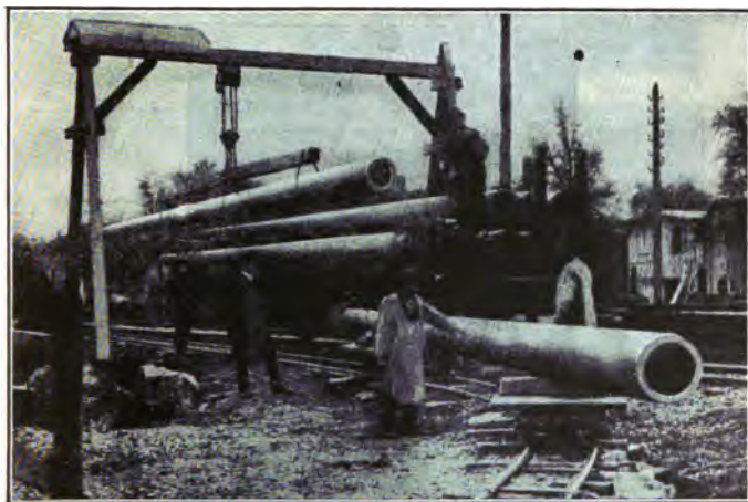
FIG. 38.—Hollow concrete poles manufactured by the Centrifugal Process.
