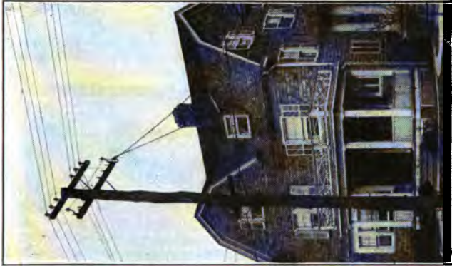
FIG. 417.—Consumers' service duplex cable.
