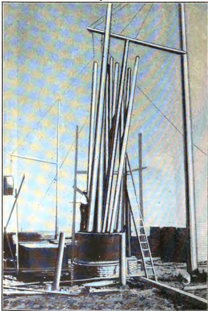
FIG. 348.—Butt treatment of poles in open tank.
