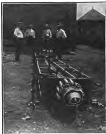
FIG. 39.—Hand-made hollow concrete pole (collapsible core.)
