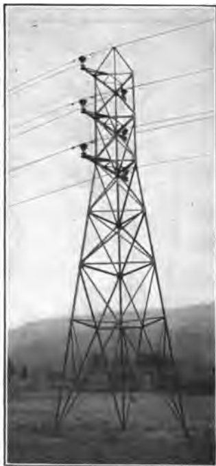
FIG. 59.—Double circuit steel tower, 40 feet high.
