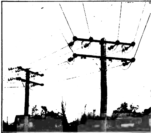
FIG. 422.—Turning a 90° bend on two poles.
