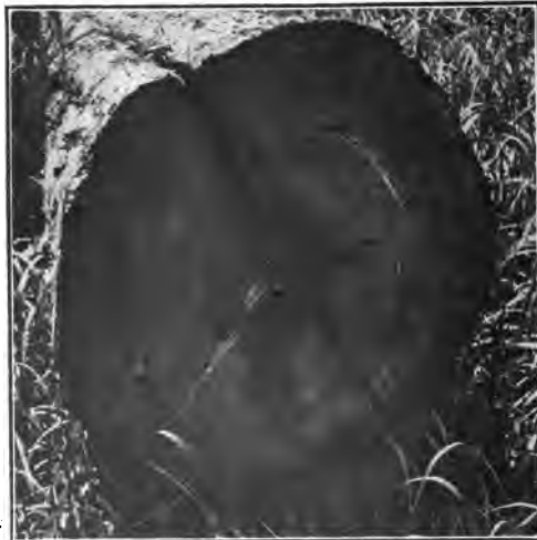
FIG. 26.—Checks and Butt Rot in Eastern White Cedar Pole.
