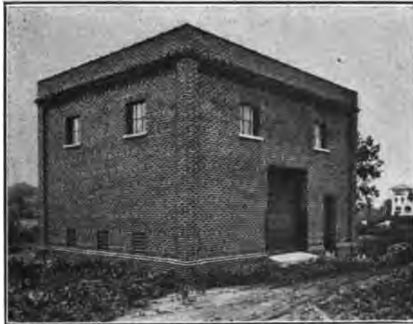
FIG. 4—EXTERIOR VIEW OF POLK BOULEVARD AUTOMATIC SUBSTATION CONTAINING 500-Kw. 600-VOLT SYNCHRONOUS CONVERTER—DES MOINES CITY RAILWAY
