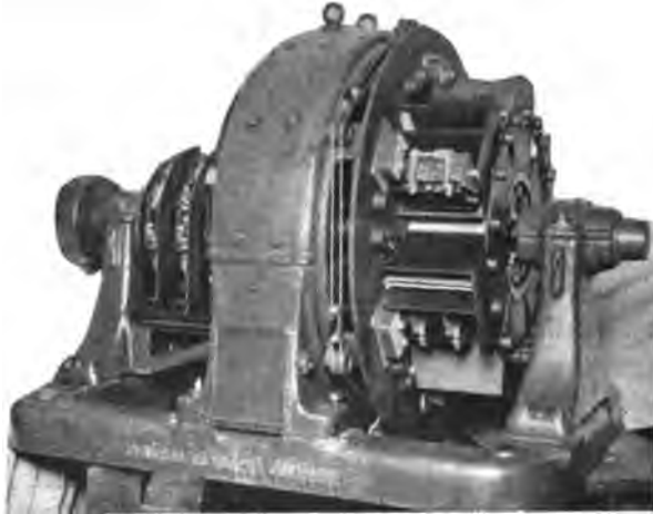
FIG. 10—500-Kw., 600/1200-VOLT 60-CYCLE SYNCHRONOUS CONVERTER EQUIPPED WITH FLASH BARRIERS
