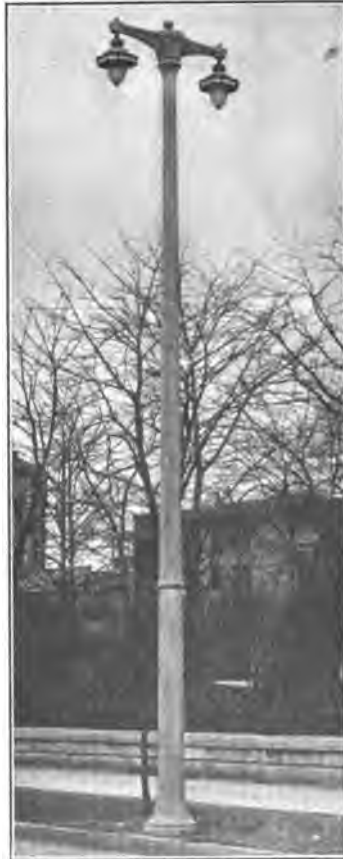
FIG. 9—30-FT. CONCRETE ROUND POST, DOUBLE BRACKET STREET-LIGHT UNIT
