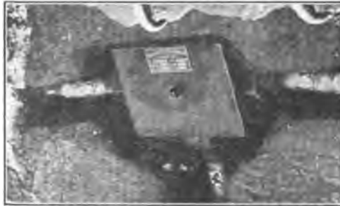
FIG. 6—INDIVIDUAL LAMP-TRANSFORMER AT BOTTOM OF STREET LIGHT POST, STEEL CASE TYPE
