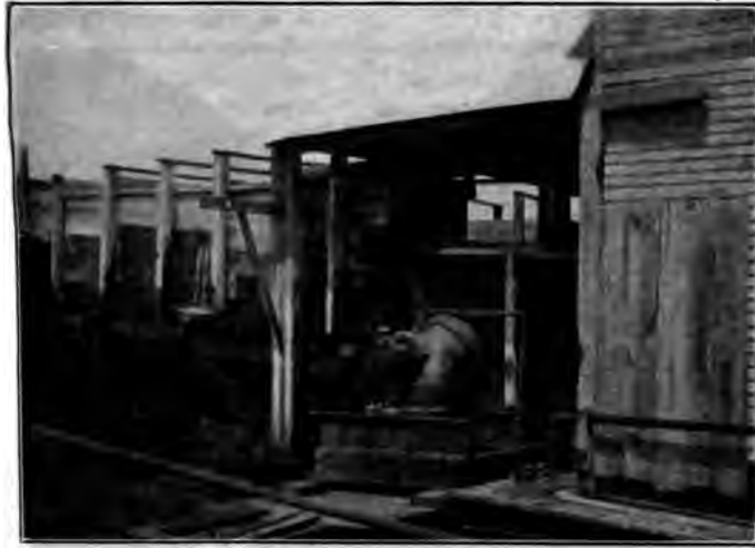
FIG. 10 VIEW OF PUMP AND FLUME, ABBOTT-DUBSON FIRST RELIEF
