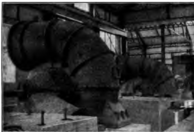
FIG. 24 76-IN. JEFFERSON-PLAQUEMINES PUMP
