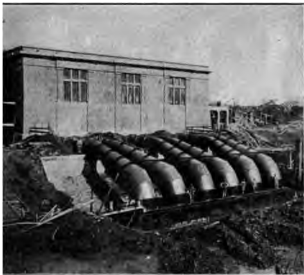
FIG. 4 EXTERIOR VIEW OF PUMPING PLANT
