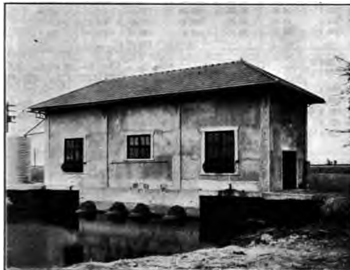
FIG. 27 PUMPING PLANT, CITRUS, LA., SHOWING SUCTION PIPES AND SUCTION BASIN
