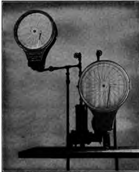
FIG. 2 MERCURY FLOAT DIFFERENTIAL GAGE WITH SEPARATE PRESSURE RECORDER
