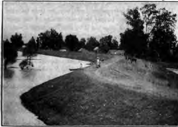
FIG. 1 MISSISSIPPI RIVER LEVEE IN LOUISIANA
