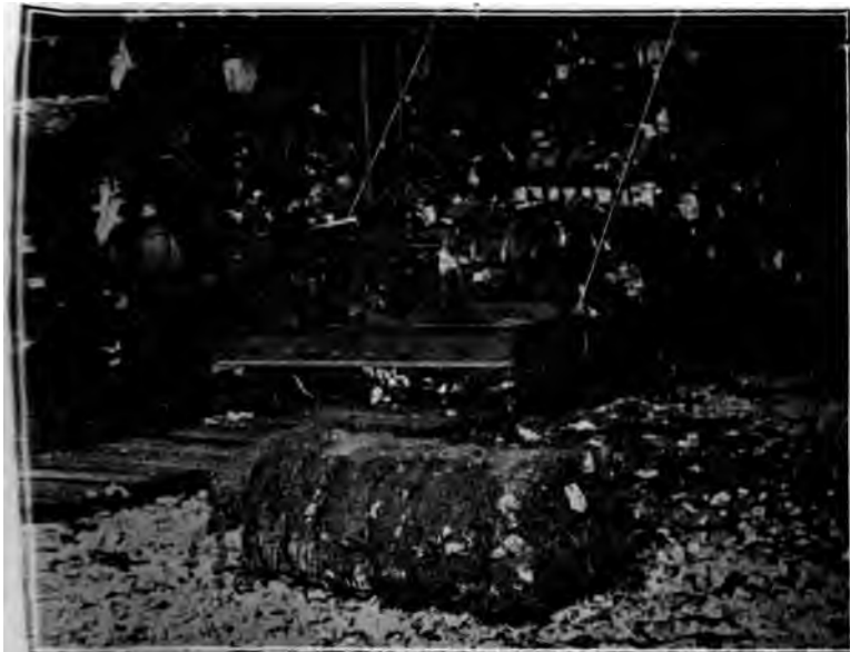
FIG. 10 AUTOMATIC GRAPPLE ABOVE COTTON BALE
