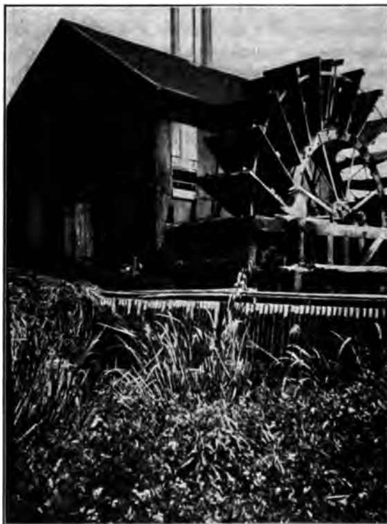
FIG. 5 DRAINAGE WHEEL, SOUTH SIDE PLANTING COMPANY
