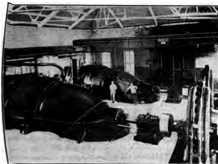
FIG. 17 12-FT. SCREW PUMPS, DRAINAGE STATION NO. 1
