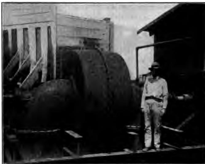
FIG. 11 IVENS PUMP AT ACADIA CANAL RELIFT
