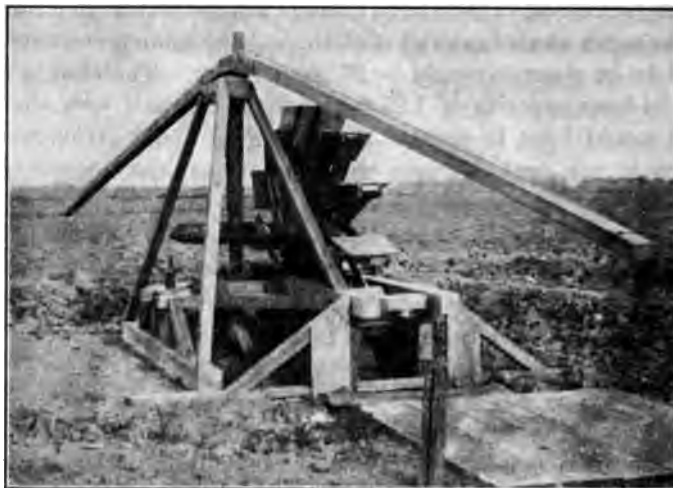
FIG. 4 SMALL DRAINAGE WHEEL
