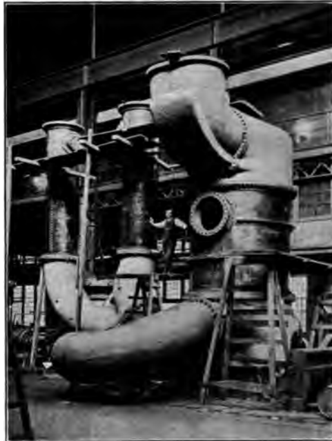
FIG. 16 GENERAL ARRANGEMENT OF SEPARATOR
