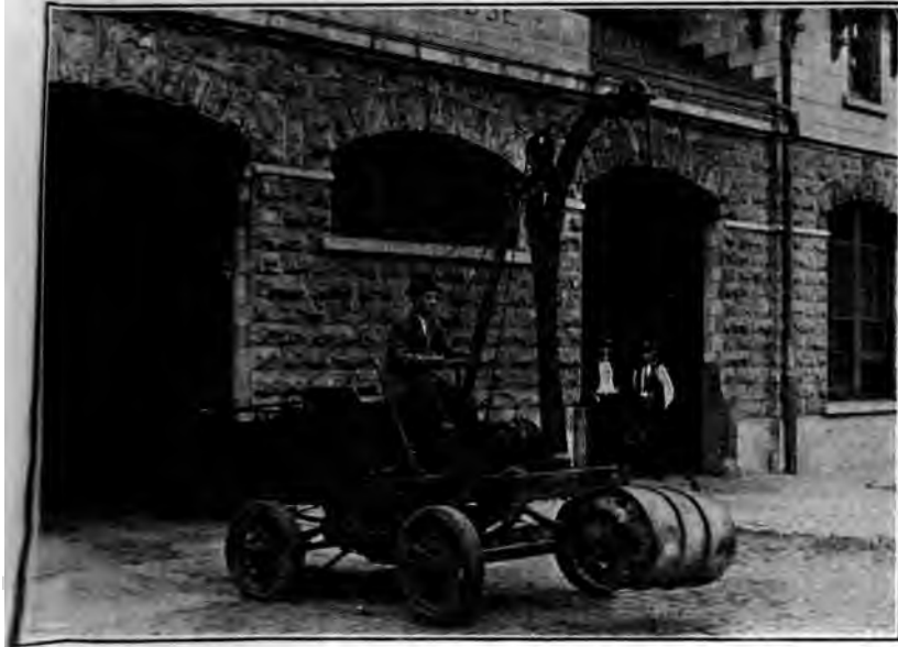
FIG. 17 STORAGE-BATTERY CRANE TRUCK
