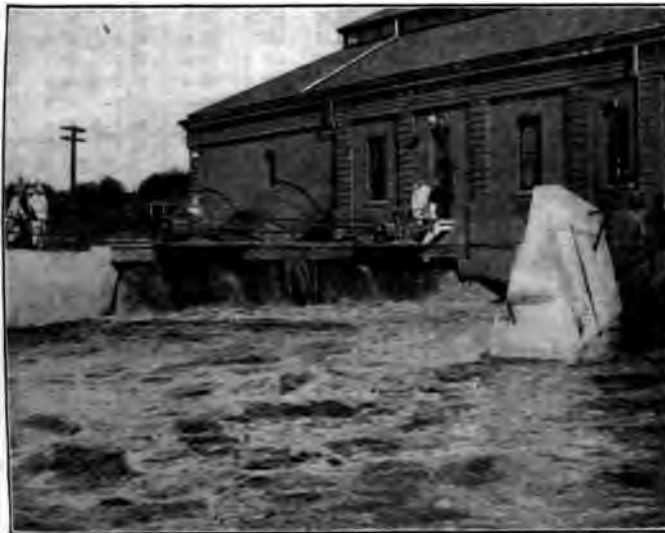
FIG. 18 DISCHARGE FROM ONE SCREW PUMP AT STATION NO. 1
