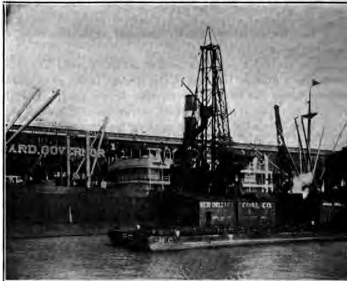
FIG. 5 TYPICAL FLOATING COAL ELEVATOR
