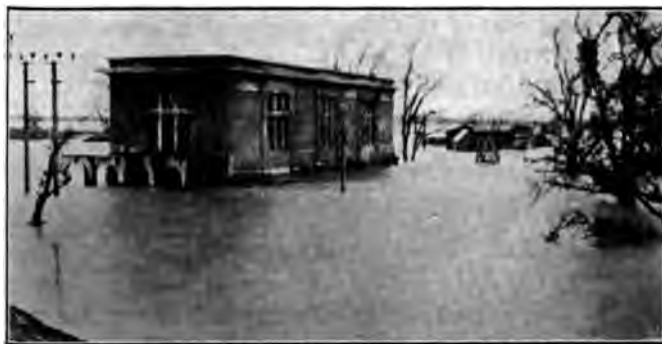
FIG. 10 GENERAL VIEW OF PUMPING PLANT
