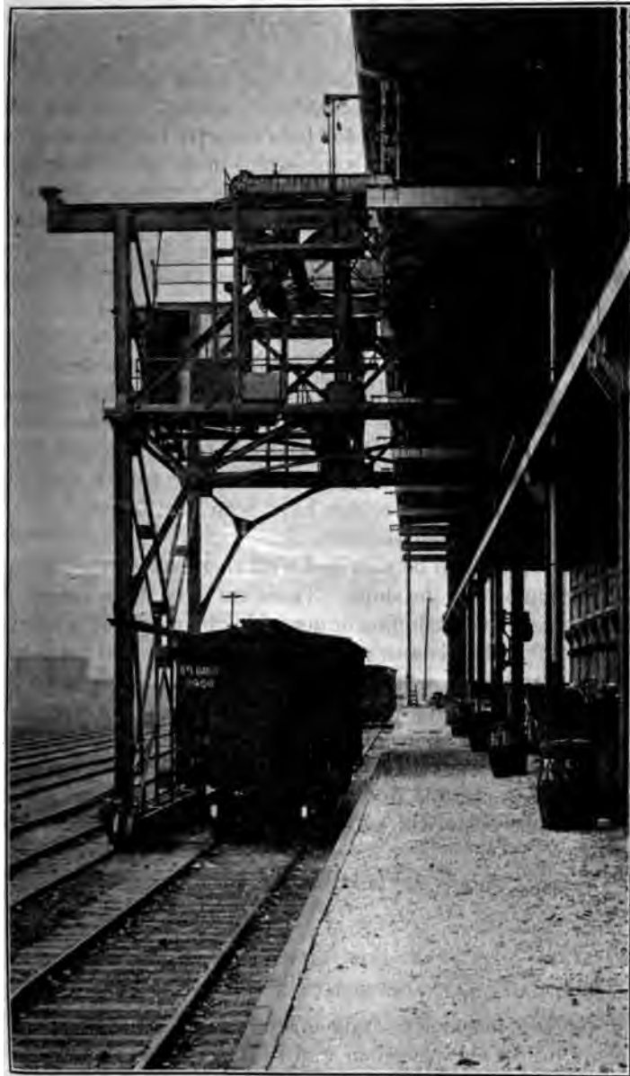
FIG. 14 TRANSFER FOR COTTON-WAREHOUSE CRANES
