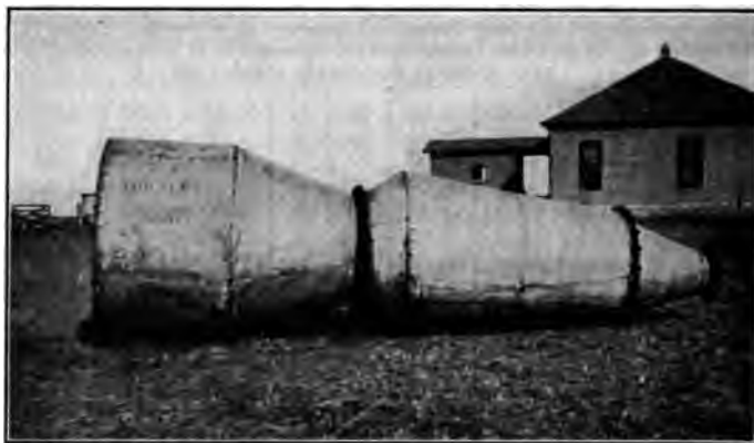
FIG. 11 OUTFLOW CHAMBER WITH SEPARATE ORIFICE PLATES
