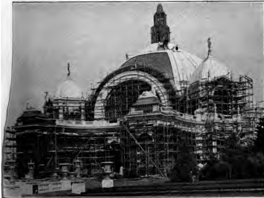
FIG. 10 FESTIVAL HALL PARTIALLY COMPLETED
