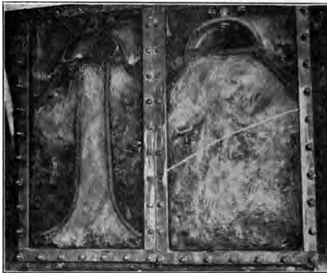
IG. 18 SHOWING FRONT HEADERS; LOAD 450 PER CENT; SETTING AS IN FIG. 8a
