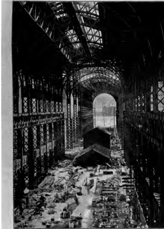
FIG. 19 FRAMING OF PALACE OF MACHINERY
