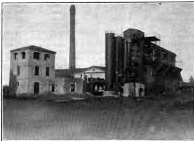
FIG. 20 PEAT POWER GAS PLANT WITH AMMONIA RECOVERY AT PONTEDERA, ITALY
