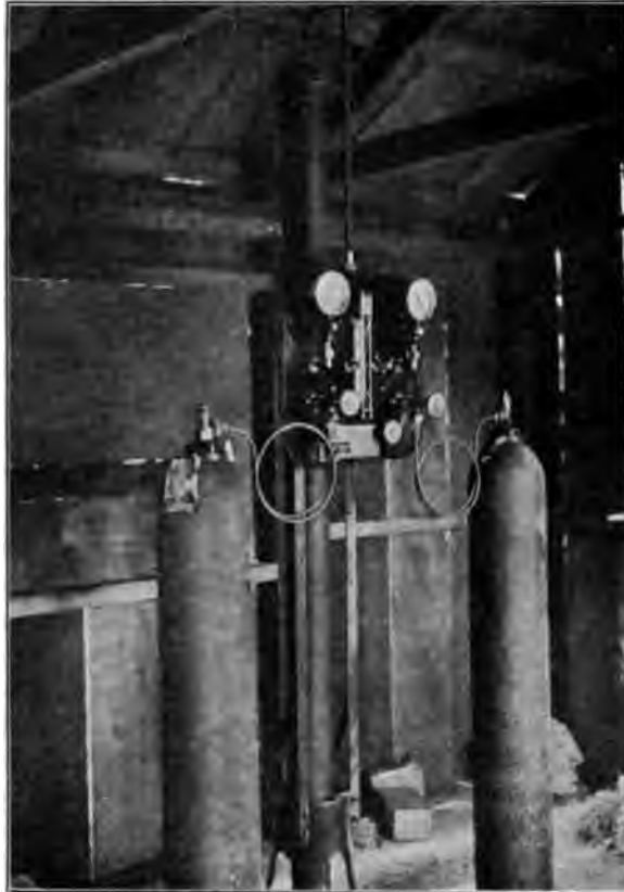
FIG. 28 APPARATUS FOR APPLYING CHLORINE TREATMENT TO WATER SUPPLY
