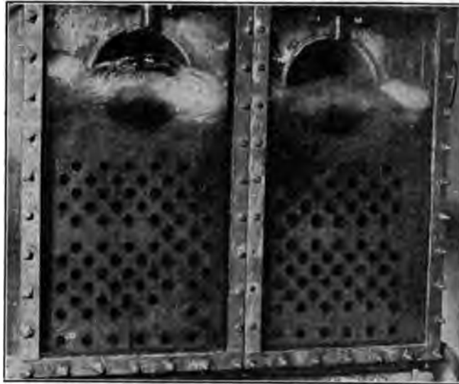
FIG. 25 REAR HEADERS, CORRESPONDING TO DESIGN OF FIG. 11 IN FRONT; LOAD 450 PER CENT; SETTING AS IN FIG. 8b
