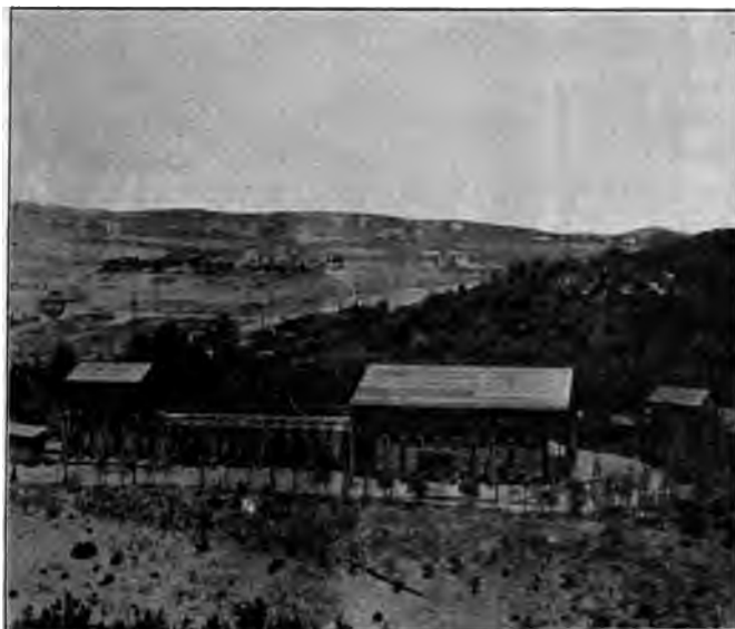
FIG. 27 FILTRATION PLANT. FILTER HOUSE IN FOREGROUND
