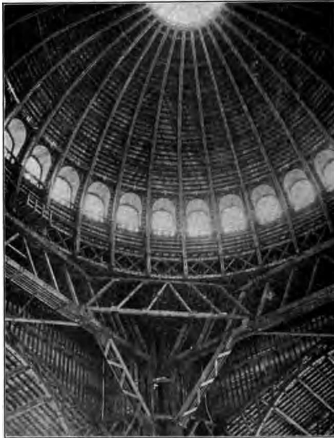
FIG. 16 INTERIOR OF DOME, MINES BUILDING
