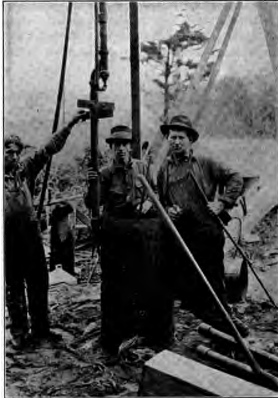
FIG. 30 PERFORATED WELL CASING AND HYDRAULIC EJECTOR
