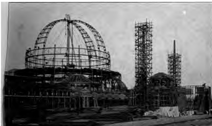
FIG. 5 HOISTING ERECTION METHOD, PALACE OF HORTICULTURE DOME
