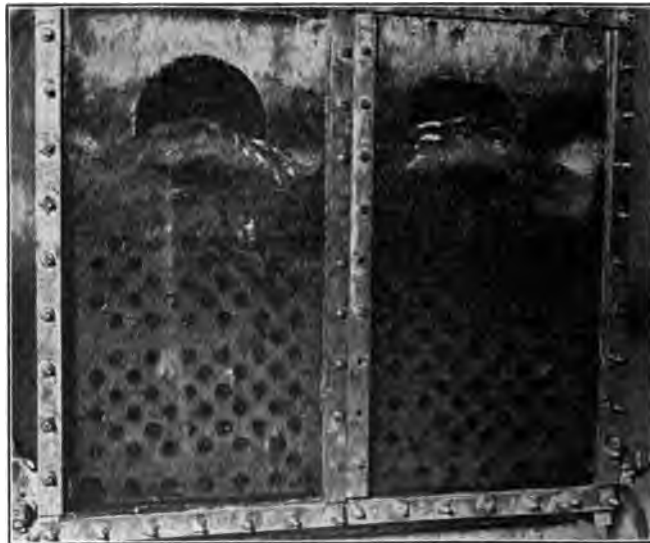
FIG. 24 REAR HEADERS CORRESPONDING TO DESIGN OF FIG. 18 IN FRONT; LOAD 300 PER CENT; SETTING AS IN FIG. 8a
