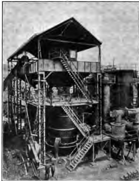
FIG. 19 5000 H.P. LYMN SYSTEM PRODUCER GAS AND BY-PRODUCT RECOVERY PLANT DURING ERECTION
