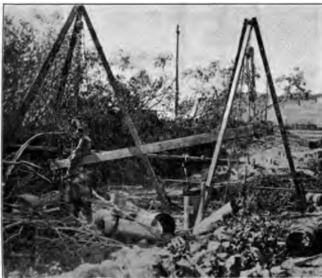
FIG. 29 RIG USED FOR DRILLING NO. 6 WELL
