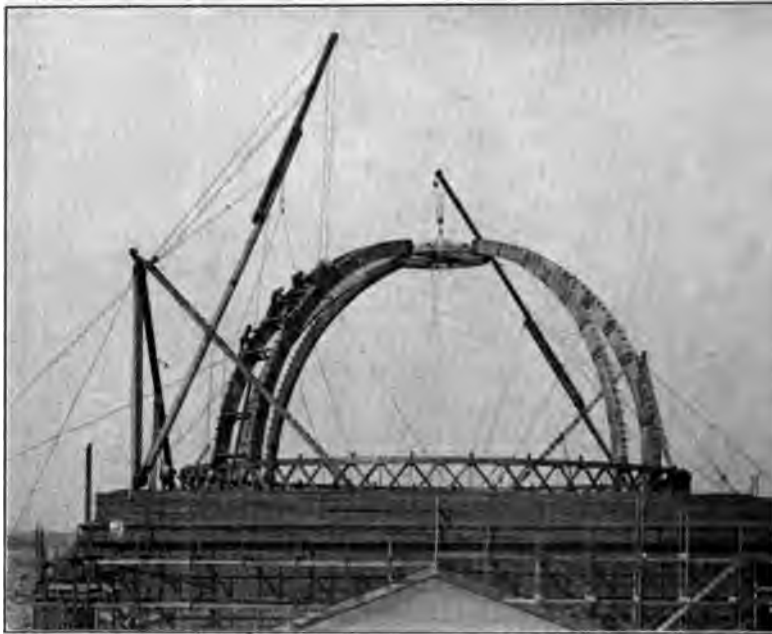
FIG. 12 TYPICAL TIMBER DOME CONSTRUCTION
