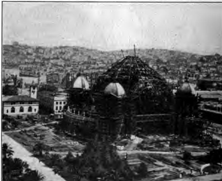
FIG. 9 DOME AND ARCHED OPENING, FESTIVAL HALL
