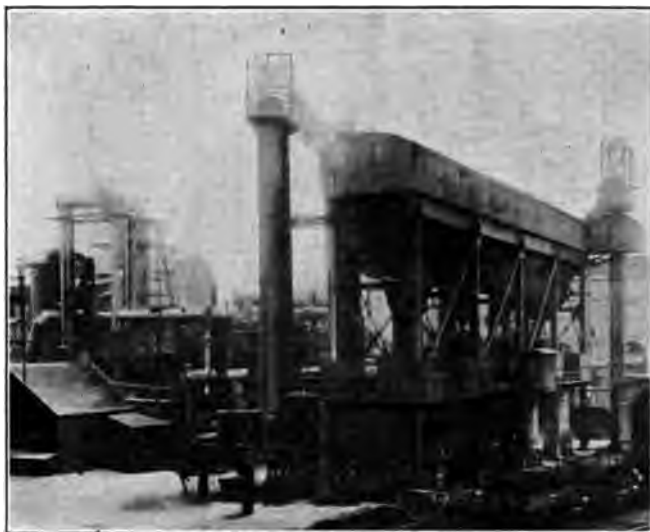
FIG. 13 8000 H.P. LYMAN SYSTEM PRODUCER GAS AND BY-PRODUCT RECOVERY PLANT
