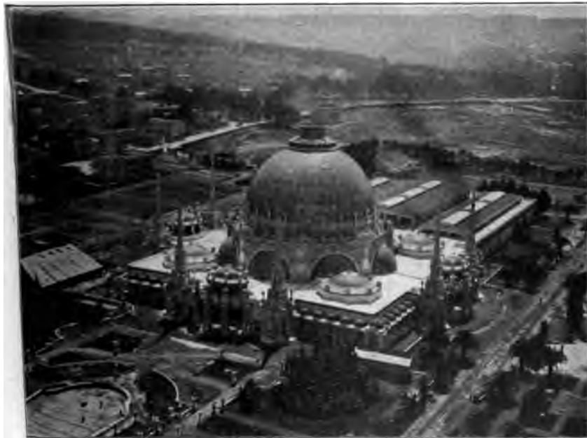
FIG. 11 COMPLETED DOME OF PALACE OF HORTICULTURE
