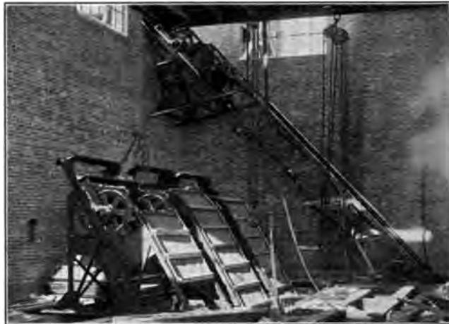
FIG. 10 INTERIOR OF SCREEN HOUSE
