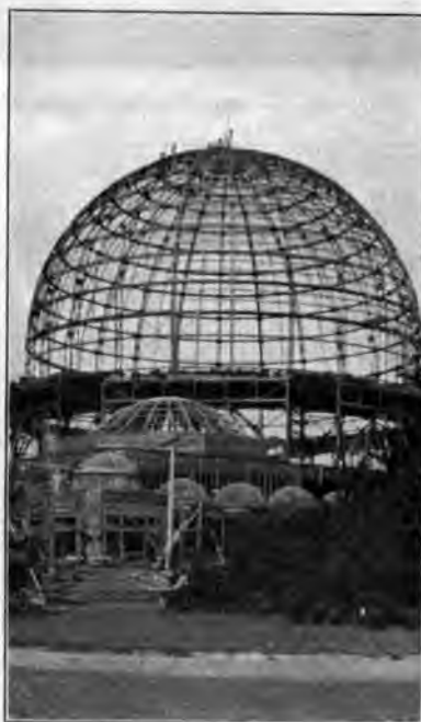
FIG. 7 STEEL DOME OF PALACE OF HORTICULTURE
