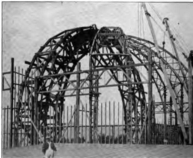
FIG. 13 FRAMING OF HALF DOME, FOOD PRODUCTS BUILDING
