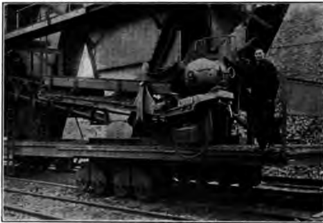
FIG. 39 MANIERRE CONVEYOR LOADER, MOUNTED ON BRIDGE PIER, CARNEGIE COAL COMPANY'S DOCK NO. 2, DULUTH, MINN.
