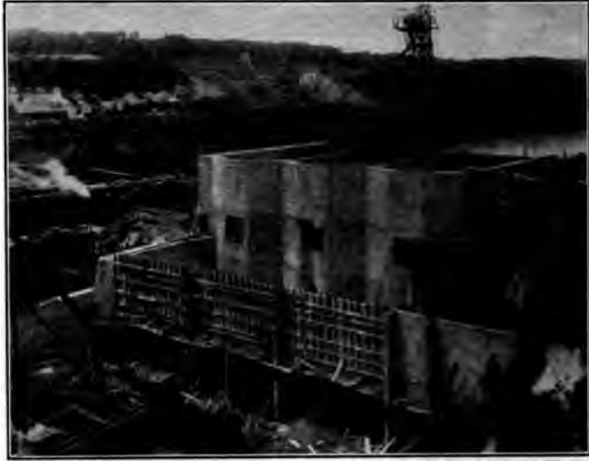
FIG. 2 CONSTRUCTION VIEW OF POWER HOUSE, JULY 1913
