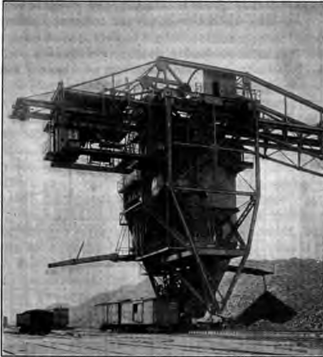
FIG. 2 SHOWING ENORMOUS STRUCTURES NOW CARRIED ON CHILLED IRON WHEELS
