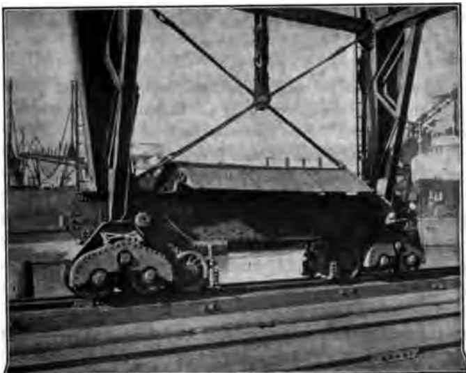
FIG. 3 DETAIL SHOWING CRANE WHEELS IN POSITION
