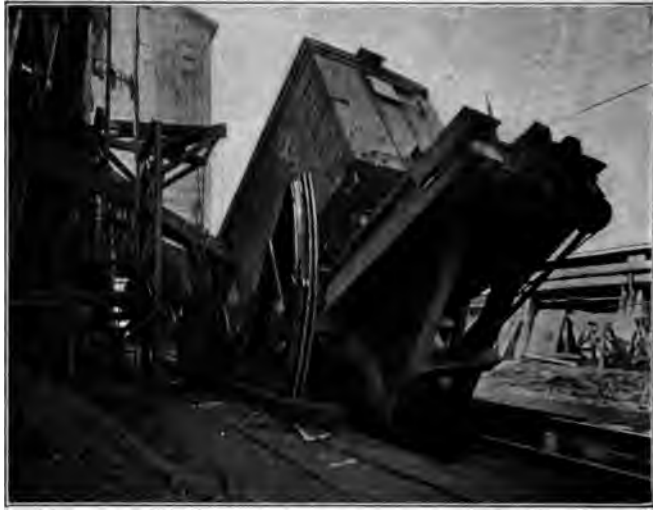
FIG. 38 SMITH TILTING BOX CAR LOADER, BUILT BY THE DODGE STORAGE COMPANY
