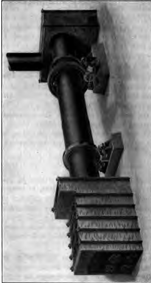
FIG. 3 GENERAL VIEW OF ROTARY DRYER WITH STATIONARY FIREBOX
