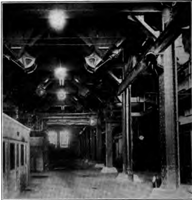
FIG. 5 VIEW UNDER COAL BUNKERS
