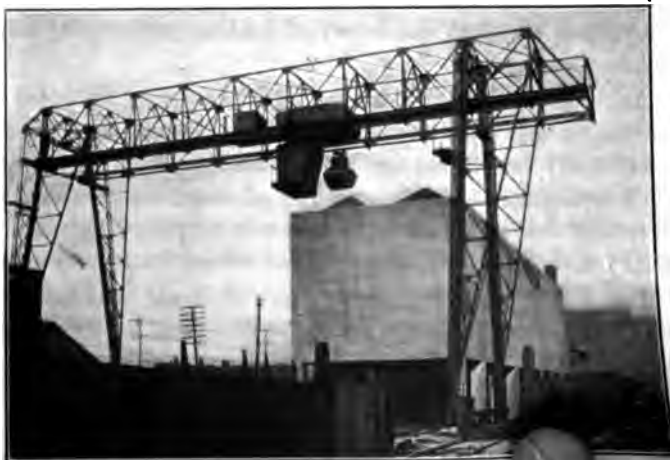
FIG. 41 McMYLER MECHANICAL PLANT FOR RETAIL YARD, PITTSBURGH COAL COMPANY'S RETAIL YARD, PITTSBURGH, PA.
