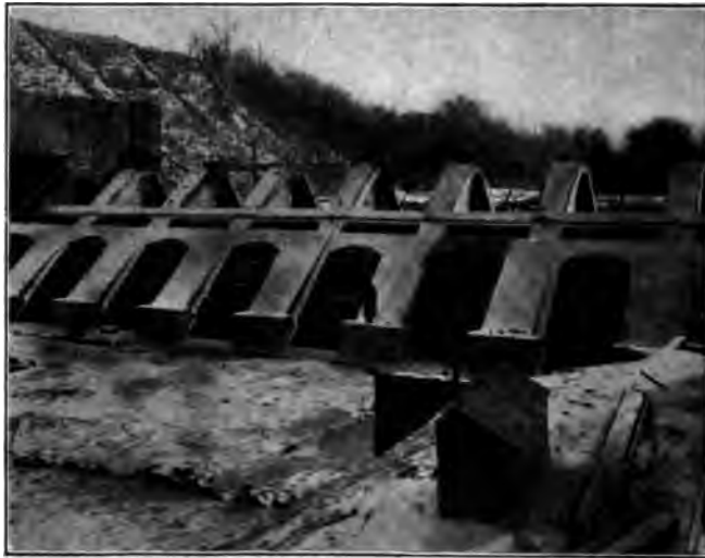
FIG. 3 VIEW OF HIGH DAM, JANUARY 1914
