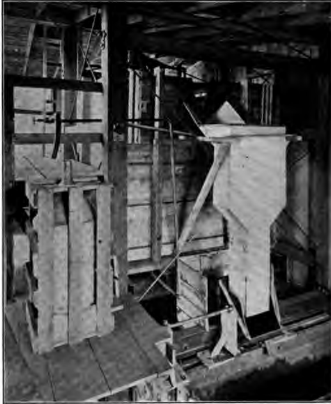
FIG. 6 STANDARD V-NOTCH USED IN TESTING PLANT
