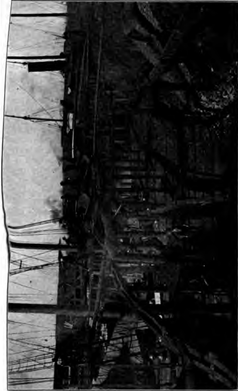
FIG. 12 EARLY METHOD OF UNLOADING COAL AND IRON ORE BY HAND SHOVELLING AND WHEELBARROW
