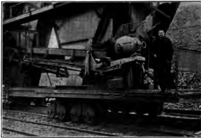
FIG. 39 MANIERRE CONVEYOR LOADER, MOUNTED ON BRIDGE PIER, CARNEGIE COAL COMPANY'S DOCK NO. 2, DULUTH, MINN.
