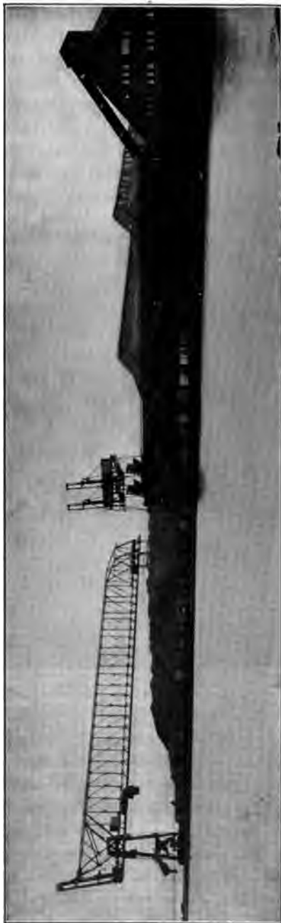
FIG. 28 NORTH WESTERN FUEL COMPANY'S DOCK NO. 1, SUPERIOR, SHOWING ANTHRACITE SECTION AND LARGEST COAL HANDLING BRIDGE INSTALLED TO DATE
