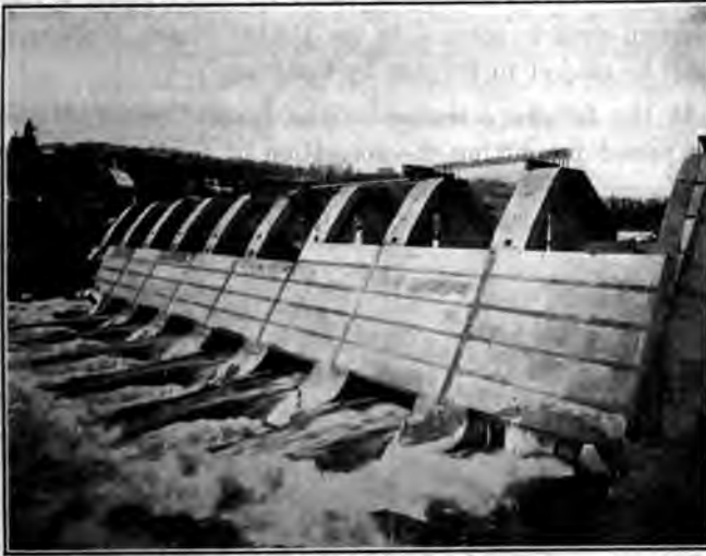
FIG. 4 VIEW OF HIGH DAM, MARCH 1914
