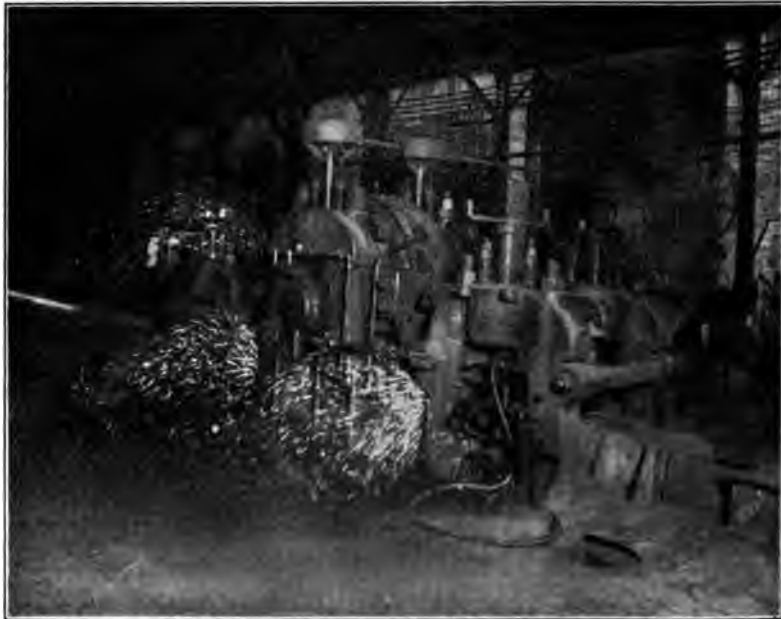
FIG. 6 HOT SAWING OR MILLING MACHINE IN OPERATION
