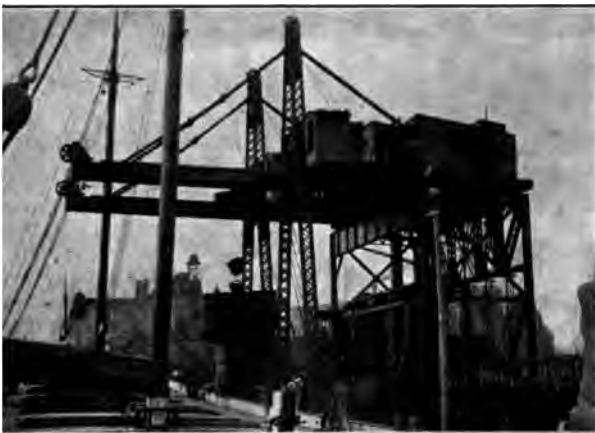
HULETT CAR DUMPER, INSTALLED ON BUFFALO, ROCHESTER AND PITTSBURGH DOCK ABOUT 1898
