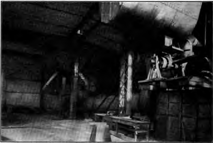
FIG. 2 VIEW FROM OPPOSITE SIDE OF MILLING BUILDING
