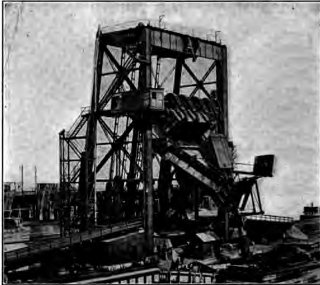
FIG. 6 McMYLER CAR DUMPER, PHILADELPHIA, PA.
