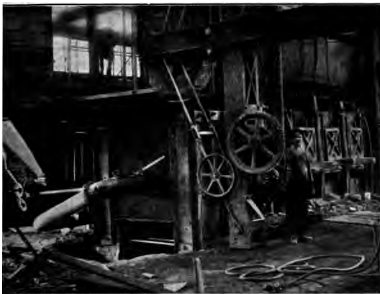
4 THREE-DOOR FURNACE WITH WASTE-HEAT BOILER, ON WHICH TESTS WERE RUN
