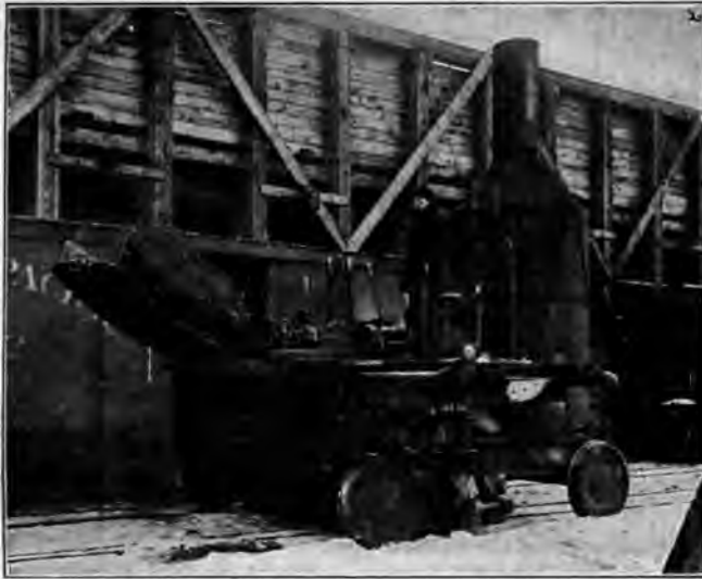
FIG. 36 OTTUMWA STEAM BOX CAR LOADER, INSTALLED ON NORTH WESTERN FUEL COMPANY'S DOCK No. 1, IN 1902. FIRST PORTABLE LOADER EVER BUILT
