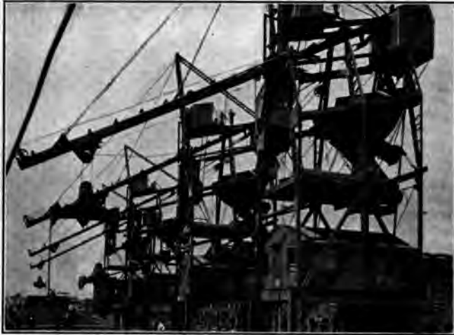
FIG. 14 BROWN HOIST TOWERS ON NORTH WESTERN FUEL COMPANY'S D No. 1, SUPERIOR, IN 1902. FIRST ELECTRIC DOCK
