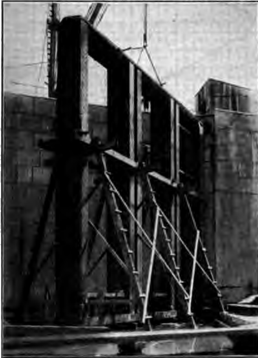
FIG. 7 LOCK AND GATE, APRIL 1913
