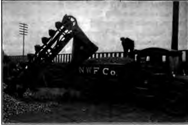
FIG. 40 SPECIALTY ENGINEERING COMPANY'S WAGON LOADER, NORTH WESTERN FUEL COMPANY'S YARD NO. 1, ST. PAUL, 1914
