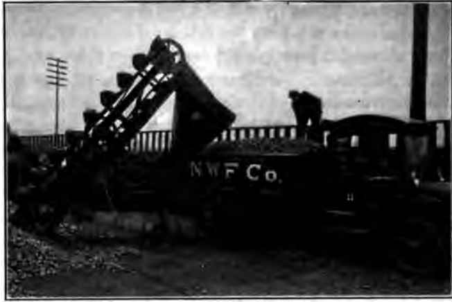
FIG. 40 SPECIALTY ENGINEERING COMPANY'S WAGON LOADER, NORTH WESTERN FUEL COMPANY'S YARD No. 1, ST. PAUL, 1914
