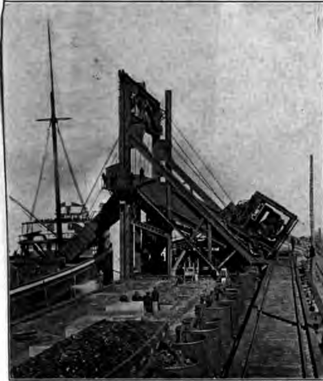
g- 7 THORNBURG CAR DUMPER, BUILT BY WEBSTER, CAMP AND LANE, 1896, AND INSTALLED AT SANDUSKY, OHIO
