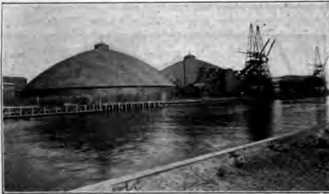
FIG. 13 DODGE COVERED ANTHRACITE STORAGE PLANT, LEHIGH VALLEY COAL SALES COMPANY, SUPERIOR, WIS.
