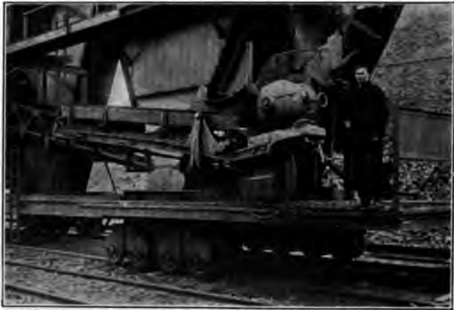
FIG. 39 MANIERRE CONVEYOR LOADER, MOUNTED ON BRIDGE PIER, CARN COAL COMPANY'S DOCK NO. 2, DULUTH, MINN.
