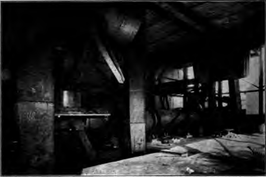
FIG. 1 MILLING BUILDING, SHOWING BINS, DRIER, PULVERIZER, ETC.
