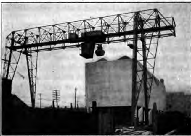
FIG. 41 MCMYLER MECHANICAL PLANT FOR RETAIL YARD, CLEVELAND AND PITTSBURGH COAL COMPANY'S RETAIL YARD, CLEVELAND, OHIO
