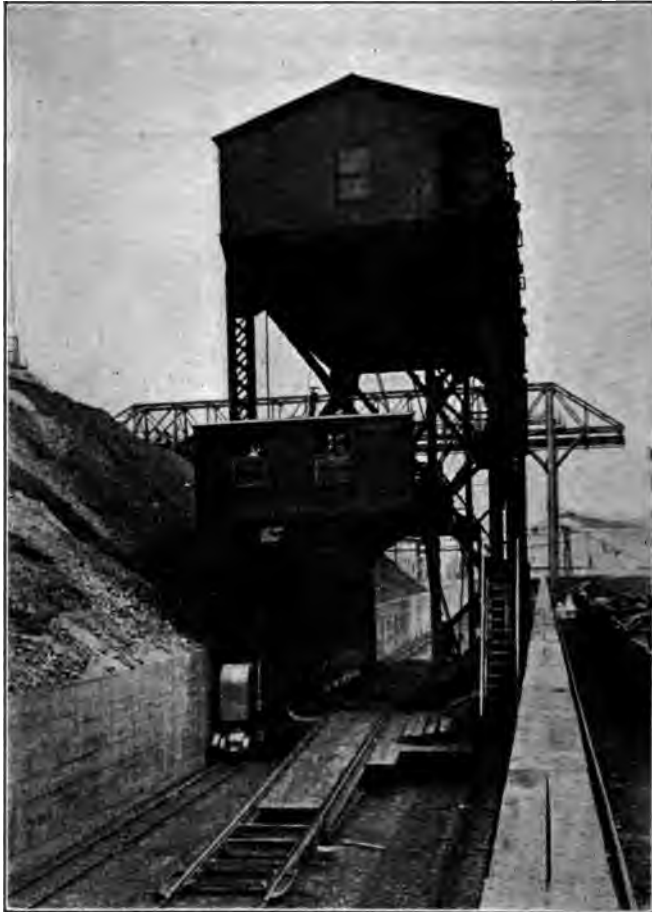
FIG. 8 HULETT TRAVERSING CAR DUMPER, BUILT BY WELLMAN-SEEVER-MOYER COMPANY FOR STOCKING IRON ORE AT PITTSBURGH STEEL COMPANY'S PLANT, MONESSEN, PA.
