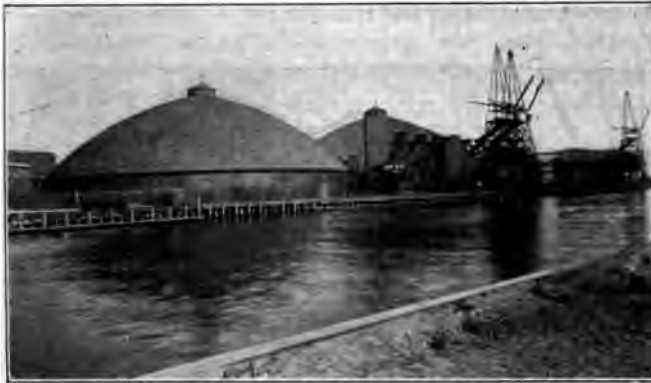
FIG. 13 DODGE COVERED ANTHRACITE STORAGE PLANT, LEHIGH VALLEY COAL SALES COMPANY, SUPERIOR, WIS.
