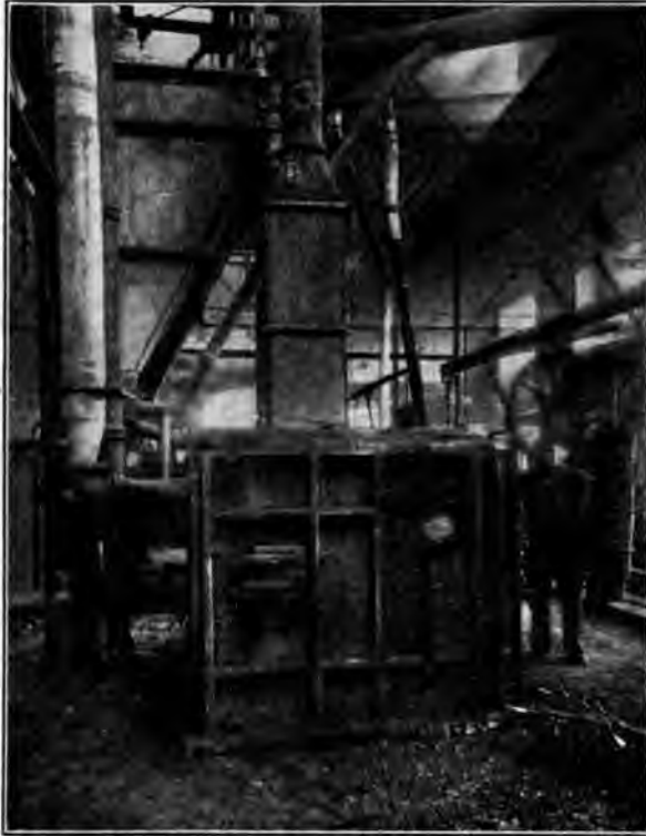
FIG. 7 FURNACE HEATING BLANKS FOR DROP FORGING, ON WHICH TESTS WERE RUN
