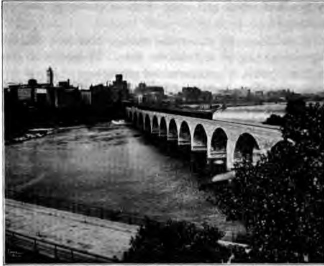
FIG. 5 MILLING DISTRICT AND FALLS FROM EAST
