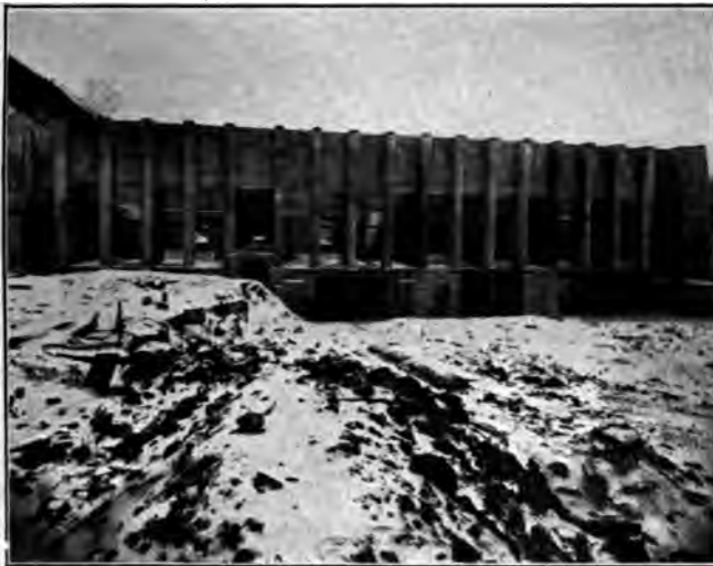
FIG. 5 VIEW OF FOREBAY, FEBRUARY 1914
