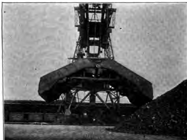
FIG. 35 HEYL AND PATTERSON 6-TON CLEAN-UP CLAM, 13 FT. 6 IN. WIDE, WITH 24-FT. REACH, INSTALLED ON NORTH WESTERN FUEL COMPANY'S No. 5 BRIDGE, DOCK No. 1, SUPERIOR, WIS.
