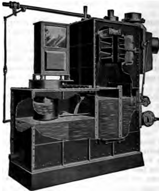
FIG. 1 V-NOTCH METER COMBINED WITH FEEDWATER HEATER
