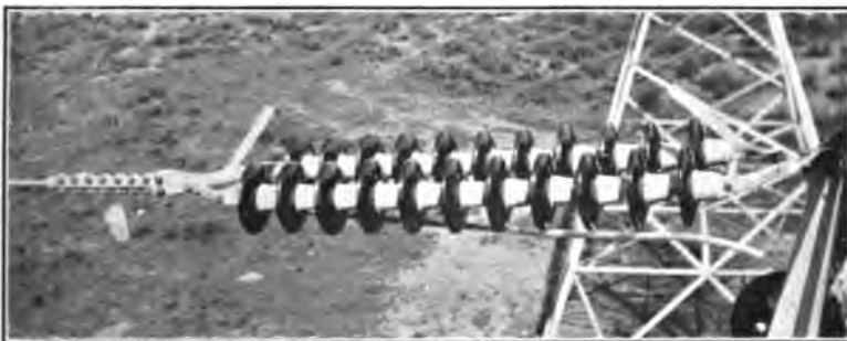
FIG. 5—150,000-VOLT STRAIN INSULATOR. [WOODBURY]
