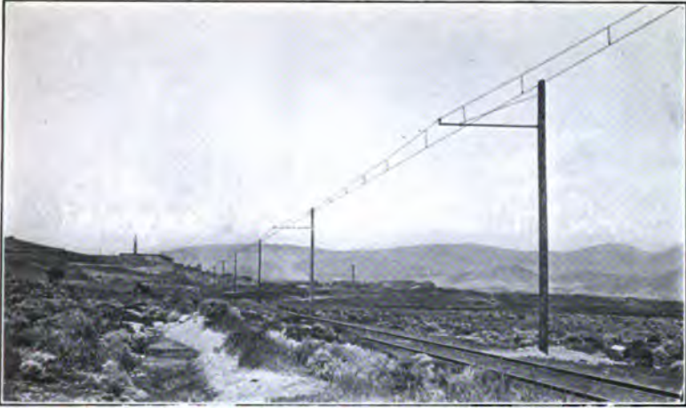
FIG. 13—BRACKET TANGENT CONSTRUCTION ON SMELTER HILL [cox]
