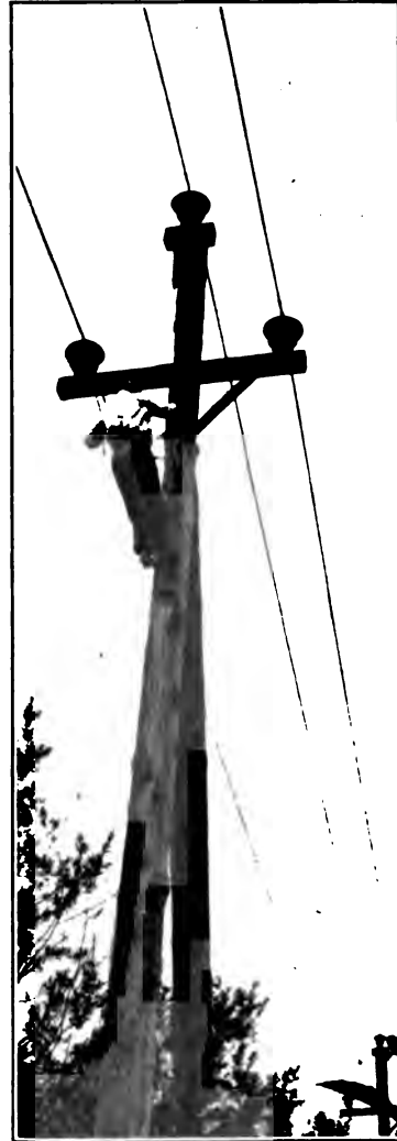
FIG. 2—SHOWING METHOD OF USING DEFECTIVE-INSULATOR DETECTING SET
