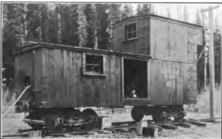
FIG. 4—PORTABLE TRANSFORMER SUBSTATION, 11,000 TO 600 VOLTS. ARMORED CABLE LEADING TO LOGGING ENGINE AT LEFT
