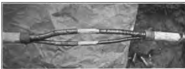
FIG. 7A—JOINTS WITH CONNECTORS SOLDERED [NIMS]
