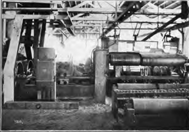
FIG. 22—200-H. P. MOTOR DIRECT-CONNECTED TO 12½ BY 84 IN. EDGER HAVING EIGHT SAWS
