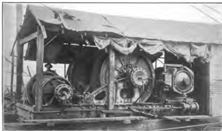
FIG. 2—ELECTRIC LOGGING OUTFIT MOUNTED ON SKIDS AT SCENE OF OPERATION [WHITNEY]
