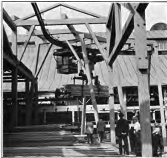
[WHITNEY] FIG. 38—MONORAIL CAR WITH LOAD FOR DRY KILN
