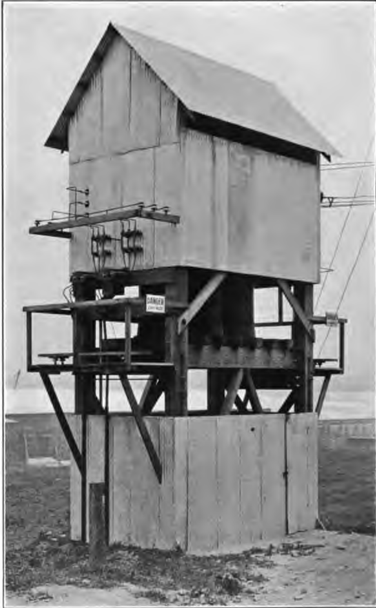
FIG. 6—RACK CARRYING THREE 333-kw., 12,000—2300-VOLT WATER-COOLED INDOOR TYPE TRANSFORMERS
