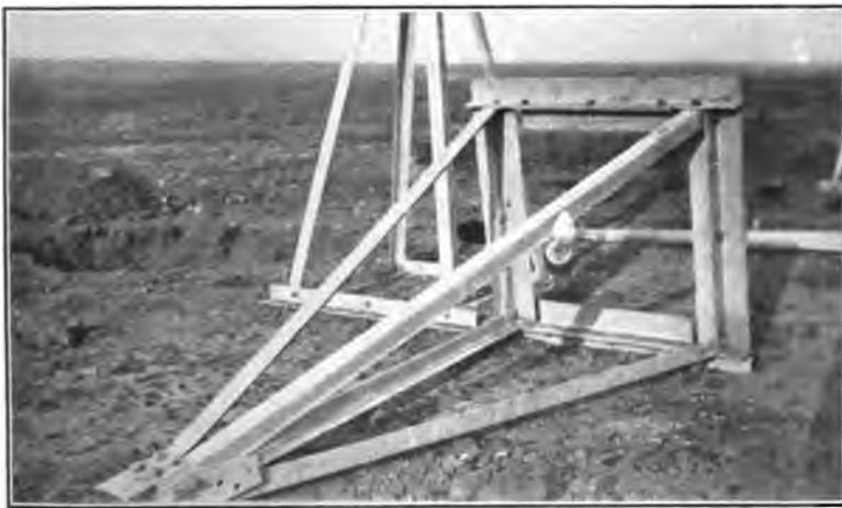
FIG. 9—STEEL FOOTING FOR STANDARD TOWER.
