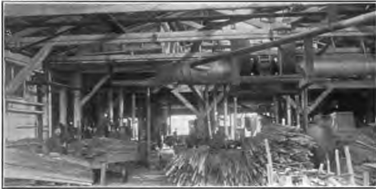
FIG. 49—DOUBLE 60-IN. EXHAUST FAN DIRECT-CONNECTED TO MOTOR
