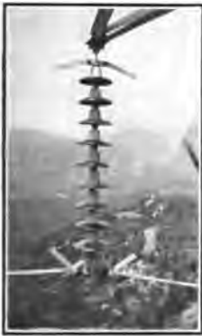
FIG. 4—150,000-VOLT SUSPENSION INSULATOR, SHOWING ARCING RODS.
