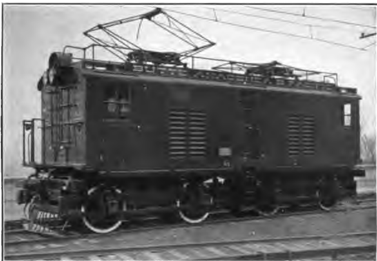
FIG. 9—EIGHTY-TON, 2400-VOLT LOCOMOTIVE [cox]
