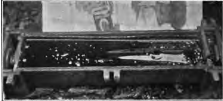
FIG. 7C—STRAIGHT JOINT BOX, PARTLY FILLED WITH BITUMEN, READY FOR COVER
