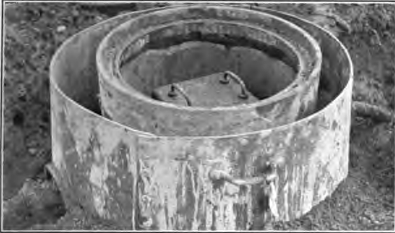
FIG. 9—SECTION BOX IN PLACE AND OUTER FORM READY FOR POURING CONCRETE
