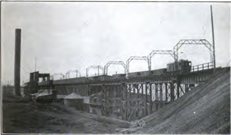
FIG. 15—STORAGE BINS AT CONCENTRATOR [cox]
