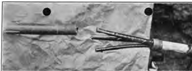
FIG. 7—CABLES SHOWING ONE END READY FOR JOINT [NIMS]
