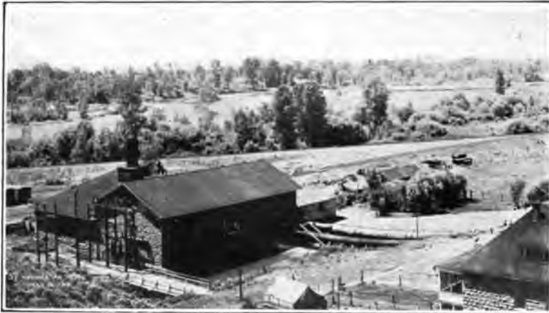
FIG. 8—NATCHES POWER HOUSE.
