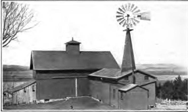
FIG. 29—THIS WINDMILL DRIVES A DYNAMO WHICH FURNISHES [BATES] CURRENT FOR TWENTY-FOUR TUNGSTEN LAMPS.
