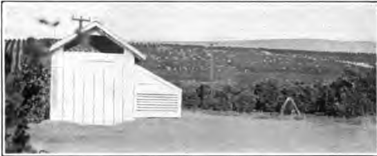
FIG. 2—800-ACRE FARM AT EXETER, CAL. • y [BATES] Pump house containing 5-h.p. electric motor, belted to 5 \frac{1}{2} -in. by 5-in. triple plunger pump with 3 \frac{1}{2} -in. suction, using 5.56 h.p.
