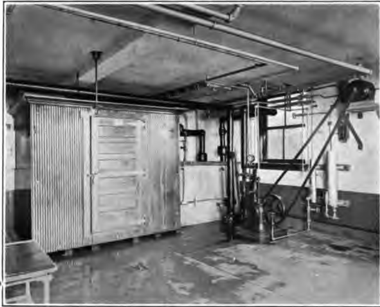
[BATES] FIG. 19— 2\frac{1}{2} -H.P. MOTOR BELTED TO AMMONIA COMPRESSOR USED FOR COOLING STORAGE REFRIGERATOR, MILK COOLER AND ICE-MAKING SET. College Farm Dairy, New Brunswick, New Jersey.
