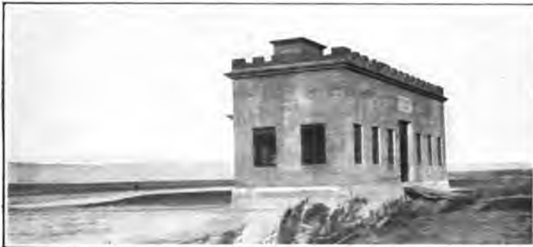
FIG. 10—AN IRRIGATION COMPANY'S PUMPING PLANT ON THE COLUMBIA RIVER.
