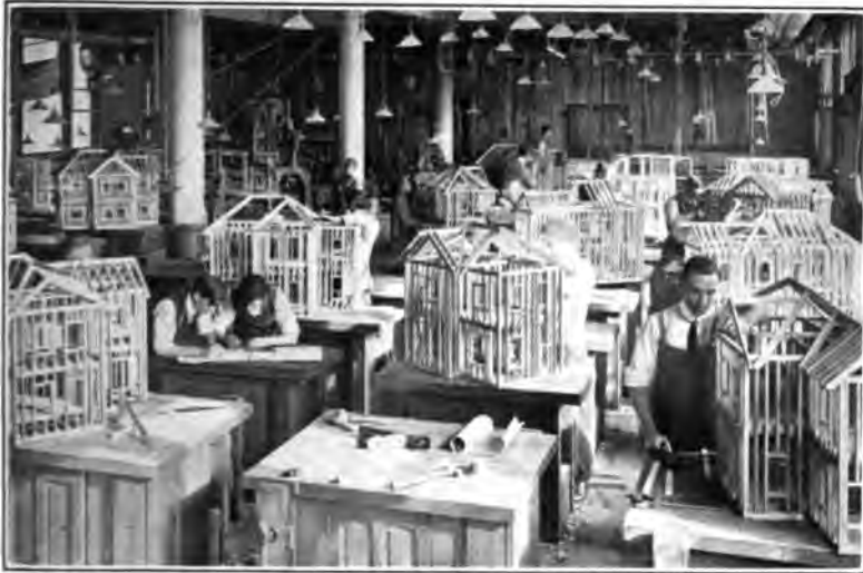
CLASS IN CARPENTRY AT PRATT INSTITUTE [SHELDON]
