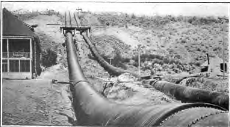
FIG. 7—PIPE LINES FROM CANAL TO NATCHES POWER HOUSE [BATES]
