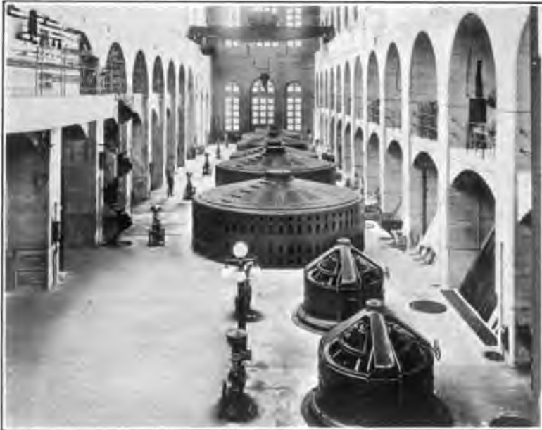
FIG. 25—POWER STATION CONTAINING TWO 400-KW., 250-VOLT WATERWHEEL-DRIVEN VERTICAL EXCITERS FOR EXCITATION OF SEVERAL LARGE ALTERNATING-CURRENT GENERATORS.
