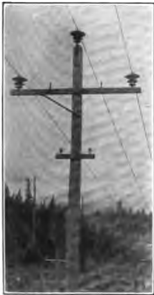
Pole-top construction on main lines. (60,000 volts)
