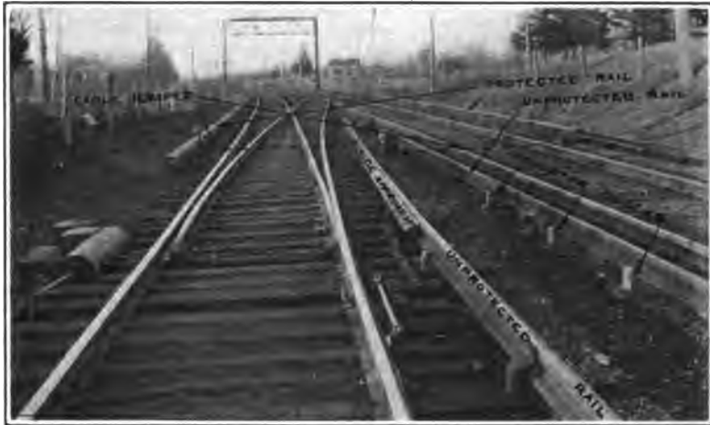
FIG. 8.—Third rail at cross-over
