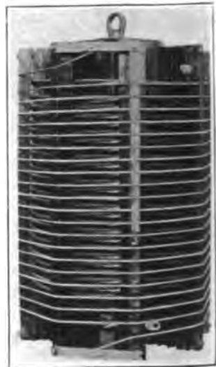
FIG. 2.—One unit of generator current-limiting reactances
