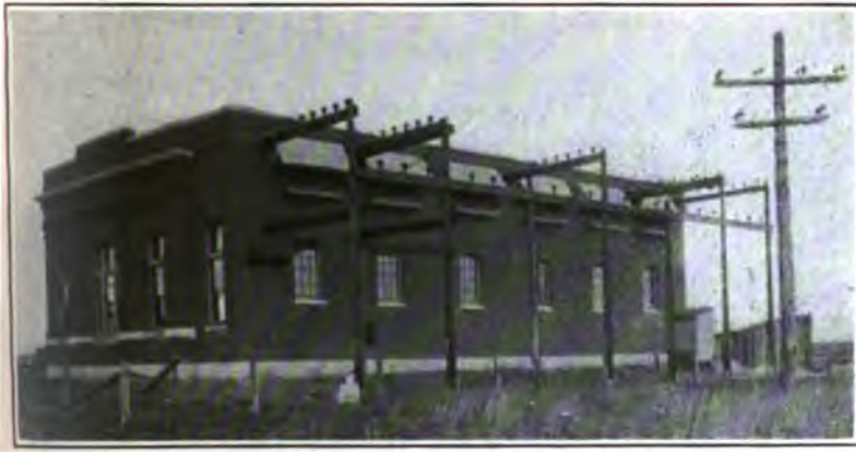
FIG. 6.—Exterior of Newfield substation
