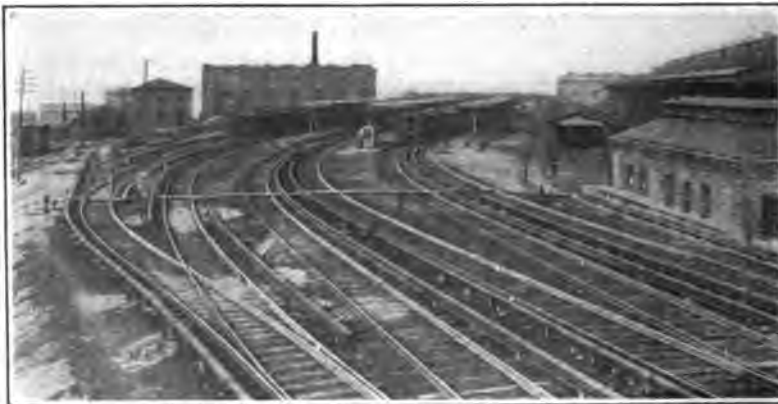
FIG. 9.—View of electrified yard at Camden terminal
