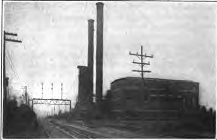
FIG. 2.—Power house at Westville, N. J.
