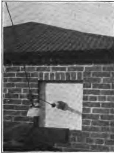
30,000-volt entrance construction
