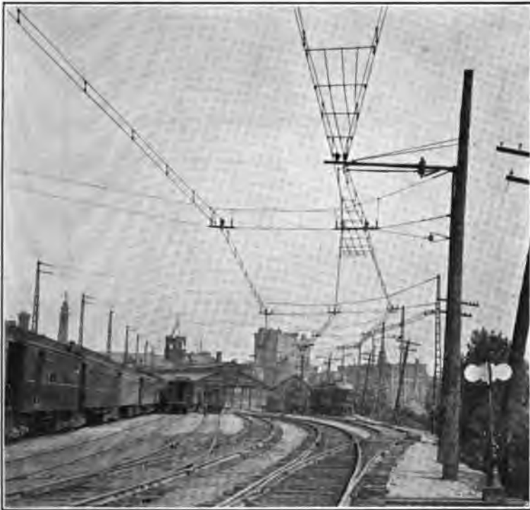
FIG. 11—Overhead construction at Rochester terminal of the Erie railroad
