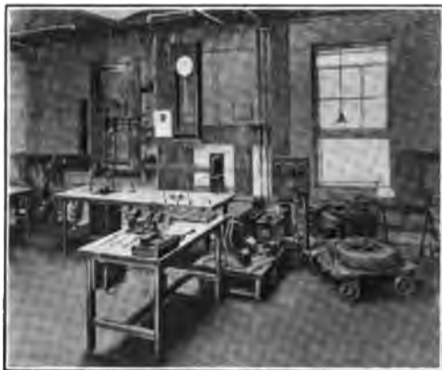
FIG. 9—Complete apparatus for testing current transformers
