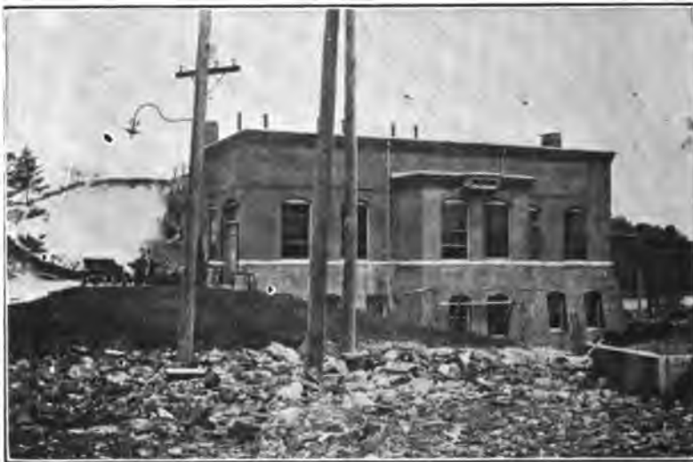
FIG. 6.—Presumpscot Electric Co. Eel Weir Falls power station
