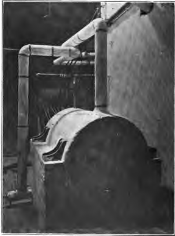
FIG. 3—Rear view of 100 kw. hot water heater
