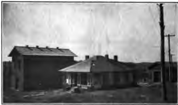
FIG. 15.—Type of sub-station
