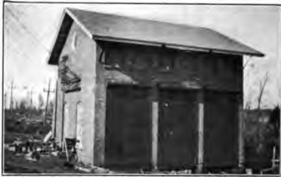
FIG. 14.—Type of sub-station
