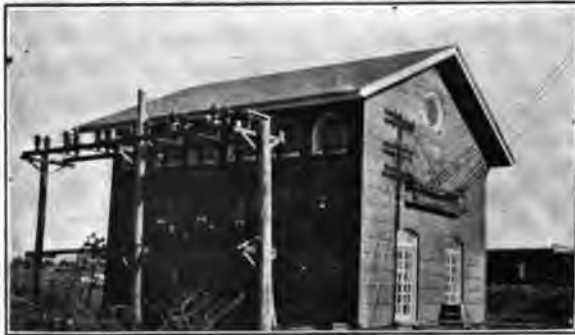
FIG. 16.—Type of sub-station
