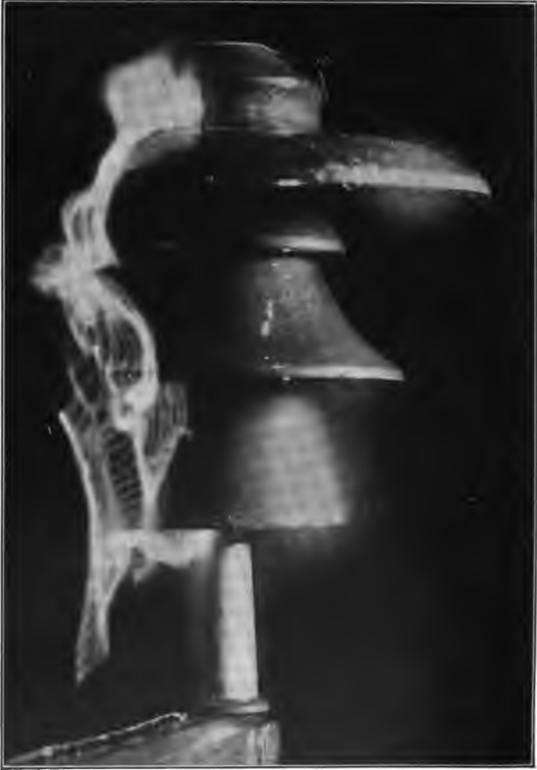
FIG. 3—Photograph of insulator flash-over, under artificial rain test
