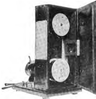
FIG. 26.—Showing Interior of Ruhmer's Photographophone.
