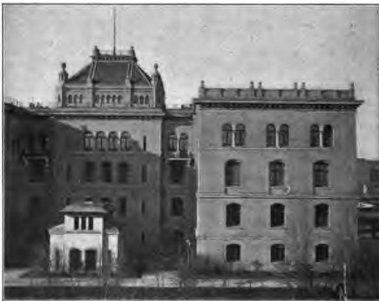
FIG. 5.—Main Building. (In part.)
