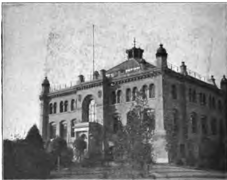
FIG. 3.—Main Building, Division I.
