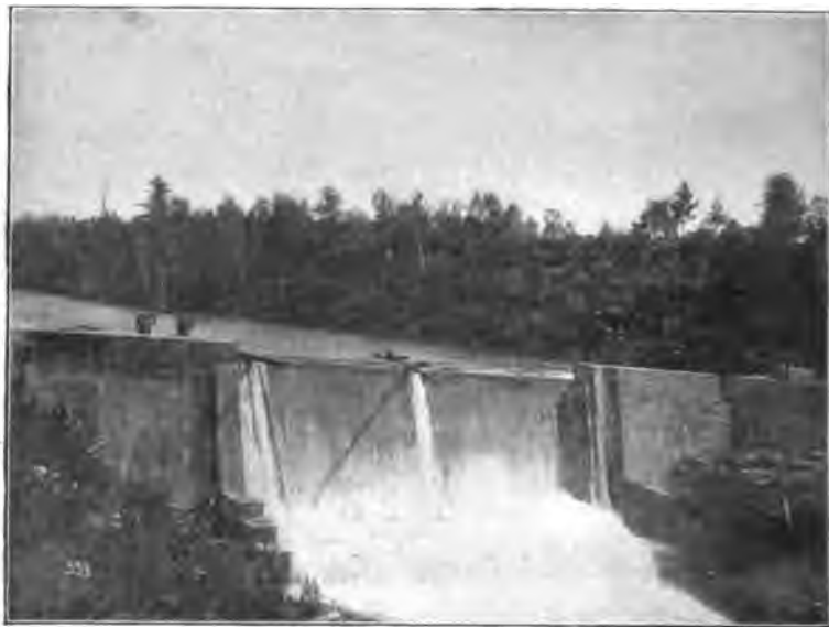
FIG. 5.—Dam and Spillway.
