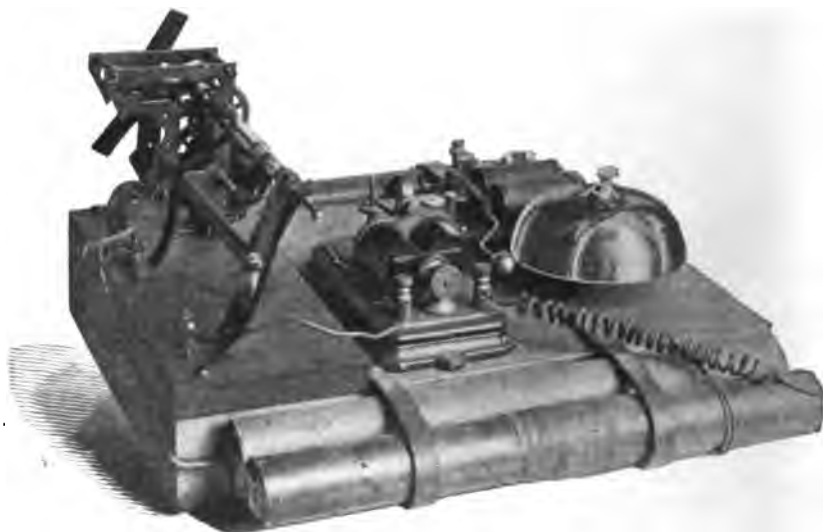
FIG. 15.—Revolving Decoherer.
