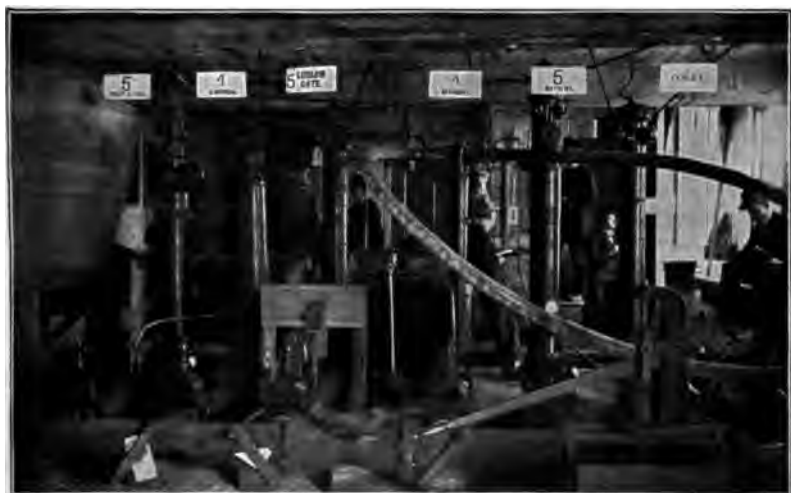
FIG. 159.—INTERIOR OF TESTING-ROOM, SHOWING HYDRAULIC TEST PUMP ON RIGHT AND WATER-HAMMER RIG TO LEFT OF CENTRE.
