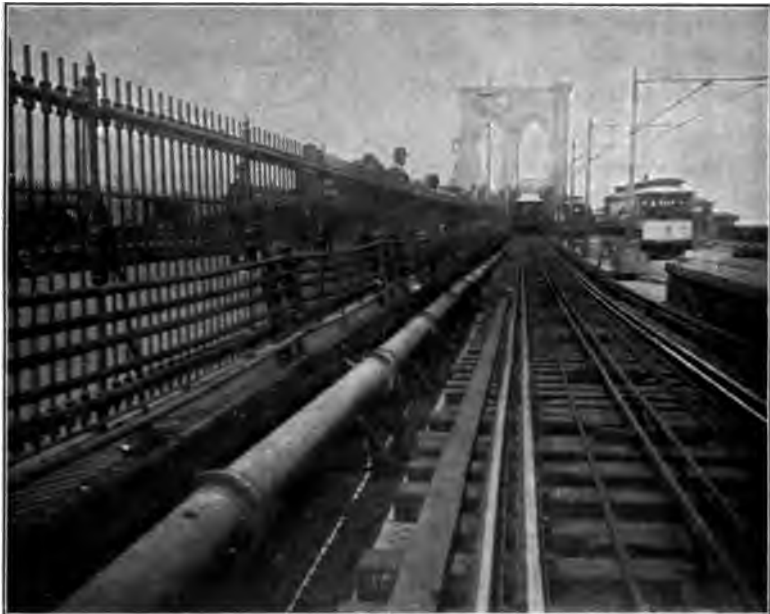
FIG. 137.—PNEUMATIC TUBES ON THE BROOKLYN APPROACH OF THE NEW YORK AND BROOKLYN BRIDGE.
