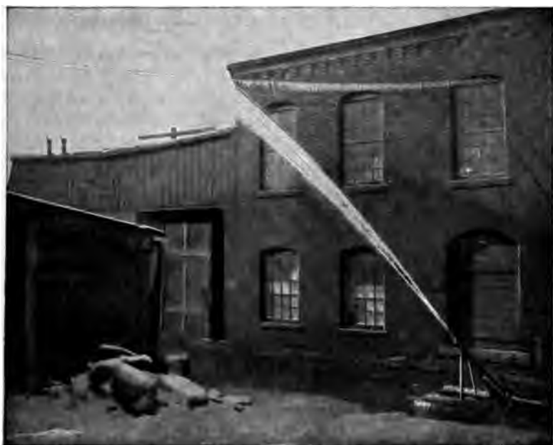
FIG. 158.—EXTERIOR OF TESTING-ROOM, SHOWING METER NOZZLE IN OPERATION.
