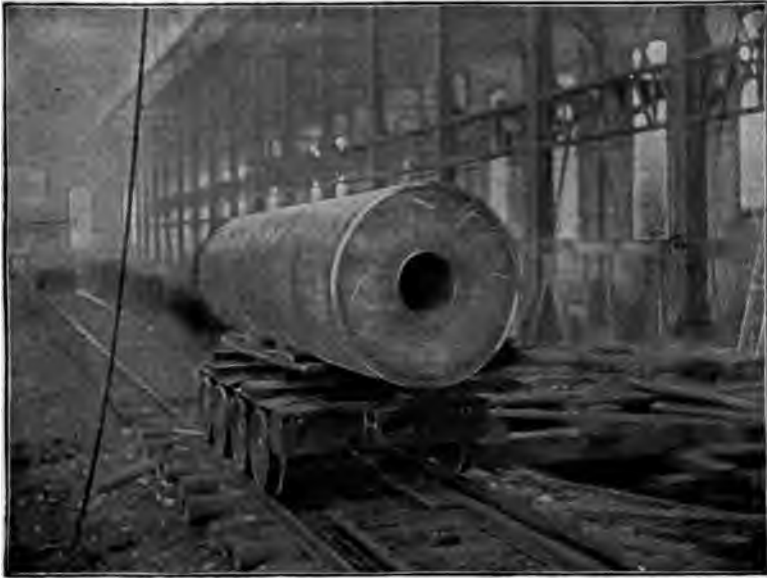
FIG. 231.—INGOT WITH 16-INCH CENTRAL HOLE AS DRILLED.
