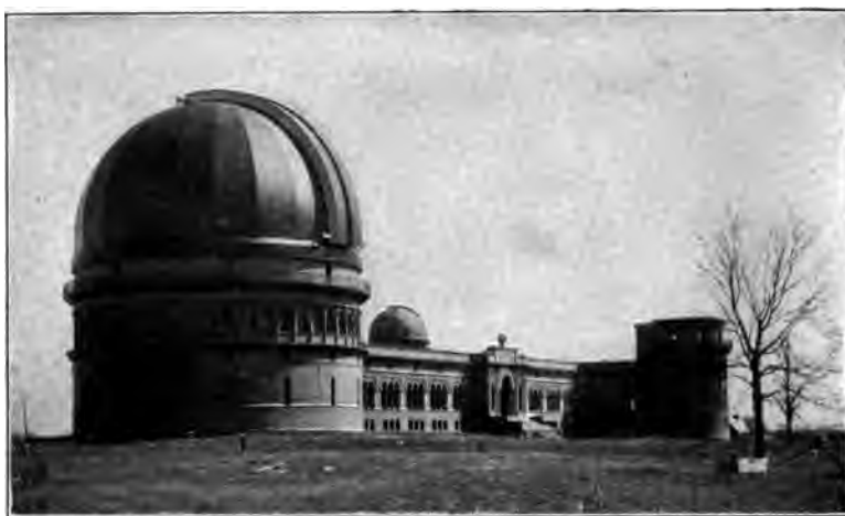
FIG. 11.—YERKES OBSERVATORY, GENEVA LAKE, WIS. LARGE DOME NINETY FEET DIAMETER.
