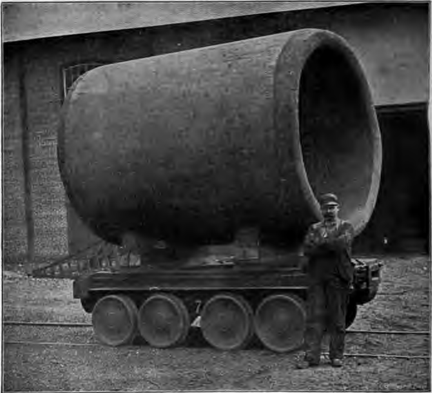
FIG. 232.—FIELD RING, AS PARTIALLY EXPANDED.
