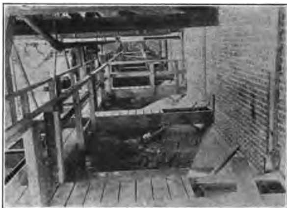
FIG. 4—MATERIAL BINS FOR DAILY CONSUMPTION
