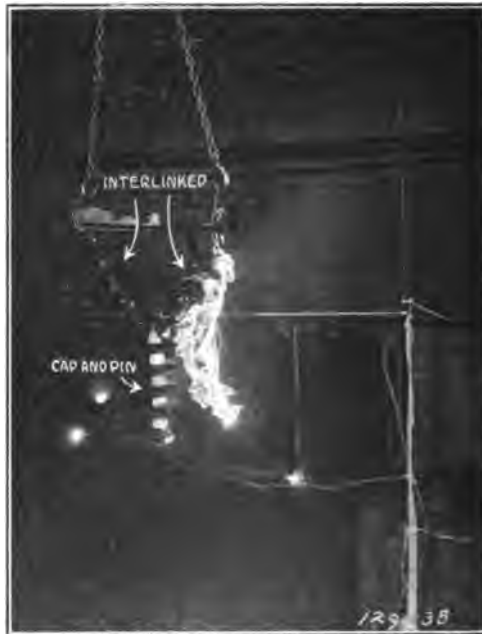
FIG. 18—60-CYCLE WET FLASH-OVER OF ASSEMBLED STRING
