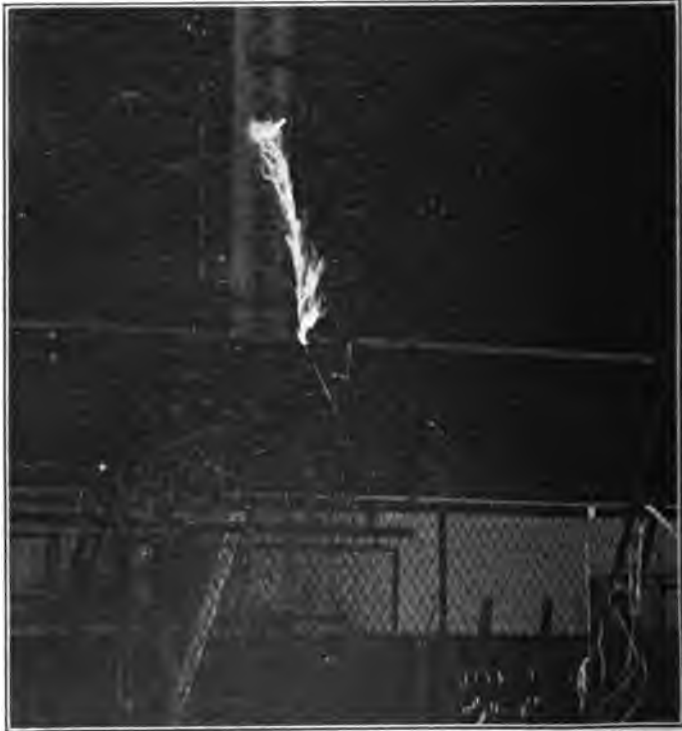
FIG. 25—WET ARC-OVER FOR ARRANGEMENT SHOWN, 508 KV. DRY ARC-OVER, 728 KV.
