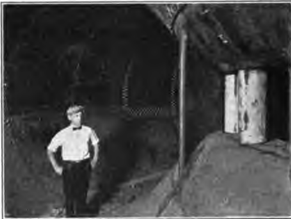
FIG. 20—INSIDE OF PLATE STEEL TURBINE CASE
