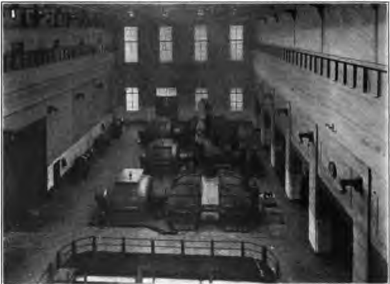
GENERAL VIEW OF TURBINE ROOM
