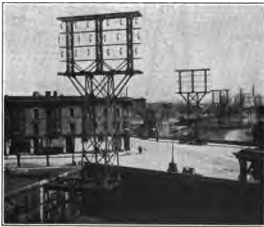
FIG. 25—TRANSMISSION LINE CROSSING STREET INTERSECTION SHOWING LONG CANTILEVER FOUNDATIONS
