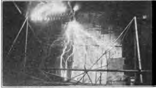
FIG. 18—HIGH-FREQUENCY ARCS WITH 2-IN. BY 12-IN. VERTICAL SHIELDS WITH INSULATOR OVER SHIELD ON TOWER SIDE
