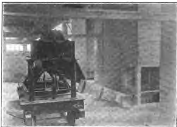
FIG. 5—METHOD OF TRANSPORTING MATERIAL TO MIXERS
