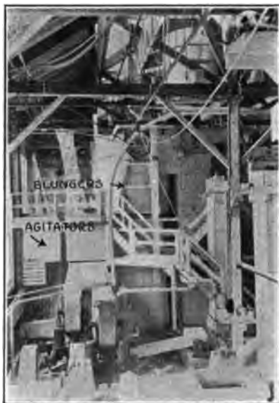
FIG. 9—GENERAL VIEW OF SECTION OF SLIP HOUSE
