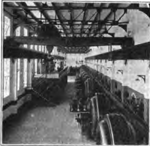
FIG. 8—INTERIOR OF STATION NO. 3 GENERATOR ROOM
