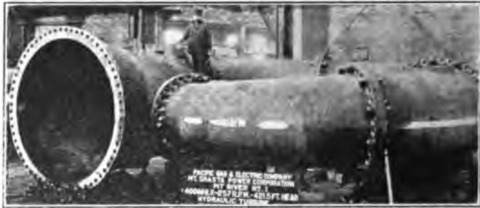
FIG. 20—CAST STEEL SPIRAL CASING
