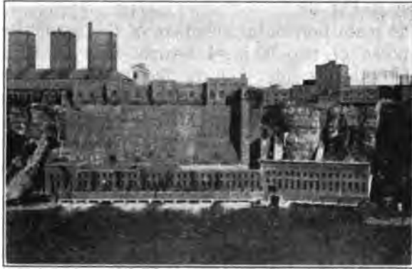
FIG. 24—VIEW OF STATION NO. 3 AND EXTENSION FROM CANADIAN SIDE OF NIAGARA RIVER
