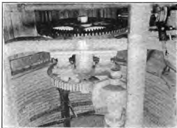
FIG. 8—VIEW OF BLUNGER DETAIL
