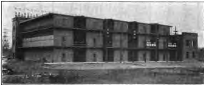
FIG. 28—ECHOTA DISTRIBUTING STATION SHOWING OUTGOING OVERHEAD LINES Most of the feeders leave the station underground
