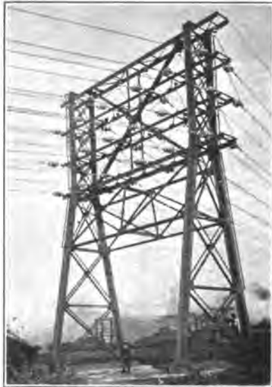
FIG. 26—PORTAL ANCHOR TOWER
