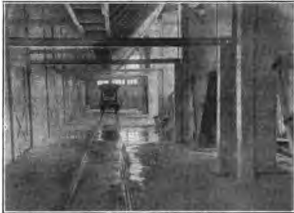
FIG. 6—MATERIAL PROPORTIONING EQUIPMENT
