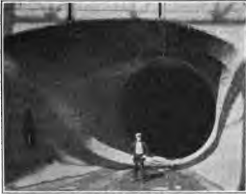
FIG. 16—BELL MOUTH AT PENSTOCK ENTRANCE
