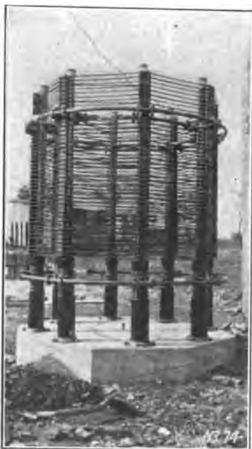
FIG. 14—OUTDOOR TUNING COIL
