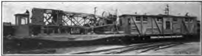
FIG. 20—RAILWAY TYPE SEARCHLIGHT EQUIPMENT, WITH POWER UNIT IN BOX CAR AND SEARCHLIGHT MOUNTED ON HINGED TOWER
