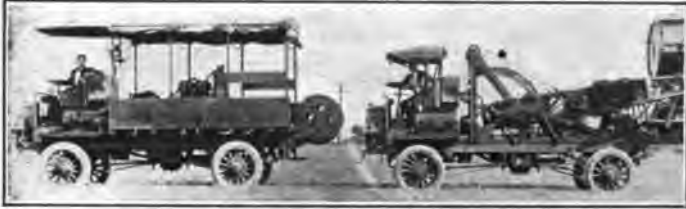
FIG. 1—TWO UNIT MOBILE SEARCHLIGHT EQUIPMENT, MOUNTED ON 3½-TON TRUCKS, SEARCHLIGHT BEING ARRANGED FOR ELEVATION BY MEANS OF AN EXTENSIBLE TOWER.
