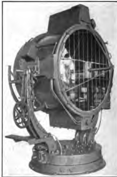
FIG. 4—60 IN. HIGH INTENSITY ARC BARREL TYPE SEARCHLIGHT, DESIGNED FOR COAST DEFENSE INSTALLATION AND USED DURING OPERATIONS OF THE 1ST AND 2ND ARMIES, A. E. F.
