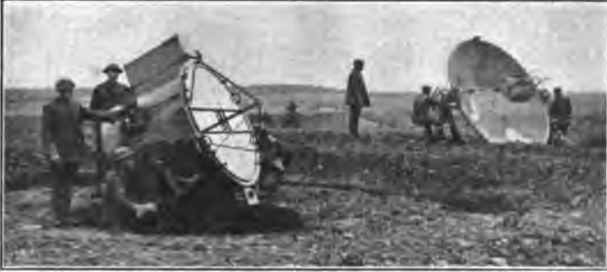
FIG. 5—A. E. F. SEARCHLIGHT EMPLACEMENT, SHOWING 60 IN. HIGH INTENSITY ARC, BARREL TYPE SEARCHLIGHT AND THREE-METER PARABOLOID.
