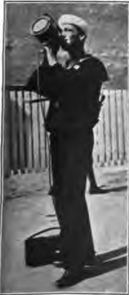
FIG. 3B—ALDIS LAMP IN SERVICE
