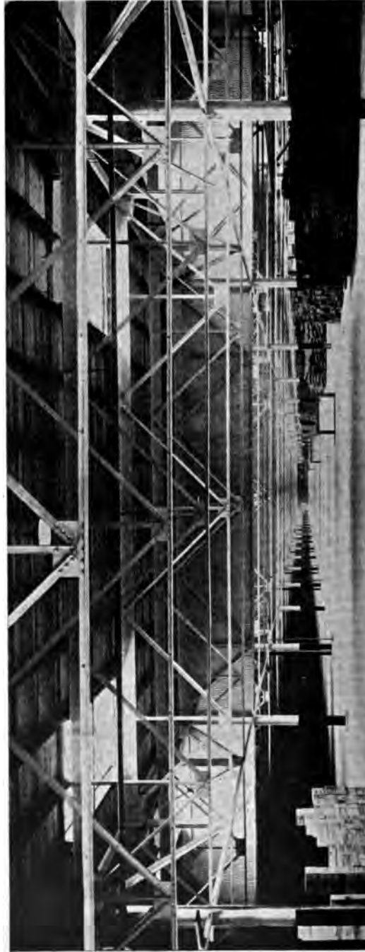
FIG. 2 SPRINKLERED PIER IN BROOKLYN, N. Y. NOTE CURTAIN BOARDS INSTALLED TO BREAK UP CEILING AREA AND BANK HEAT AT SPRINKLER HEADS
