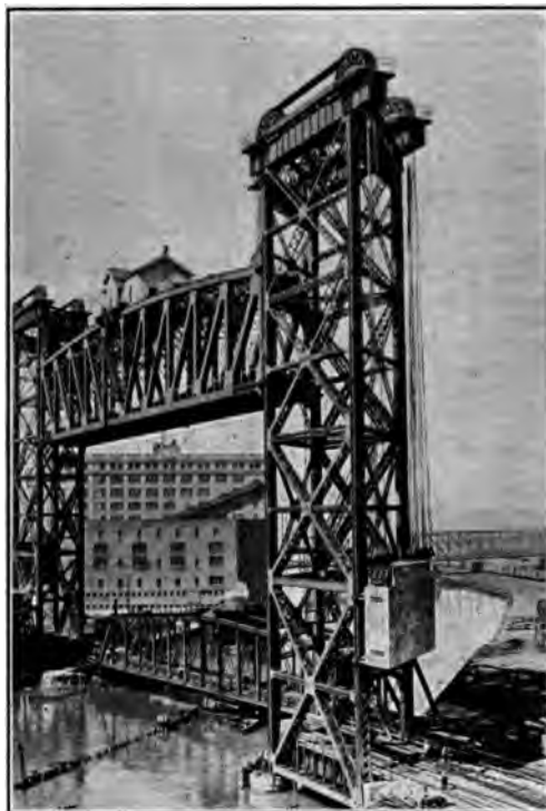
FIG. 12 BRIDGE No. 458, PENNSYLVANIA LINES, AFTER REMOVAL OF FALSEWORK
