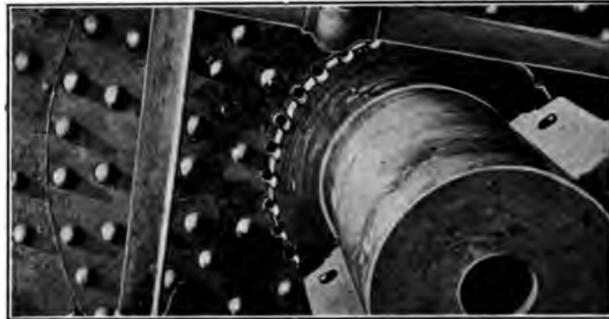
FIG. 7 REPAIRS TO HUBS OF BUILT-UP SHEAVES FOR PENNSYLVANIA LINES BRIDGES IN CHICAGO
