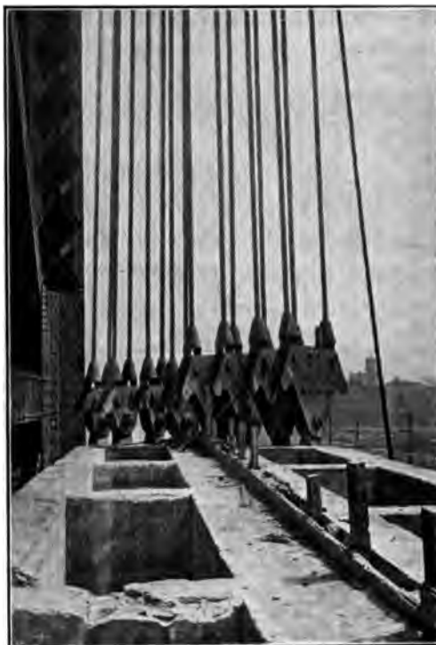
FIG. 14 EQUALIZER AND COUNTERWEIGHT, ERECTED POSITION, BRIDGE NO. 458, PENNSYLVANIA LINES
