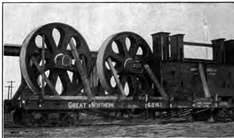
FIG. 6 TWO 12-FT. CAST-STEEL SHEAVES AND SUPPORTING GIRDER OF MISSOURI RIVER BRIDGE AT MONDAK, MONT.
