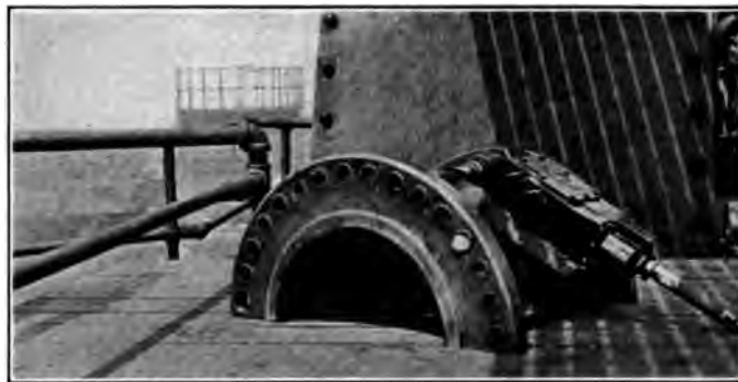
FIG. 8 CAST TEMPLET AND AIR DRILL, PENNSYLVANIA LINES BRIDGES, CHICAGO
