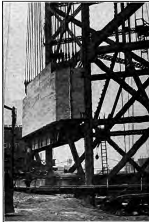
FIG. 11 COUNTERWEIGHT ON ITS FALSEWORK, BRIDGE No. 458, PENNSYLVANIA LINES
