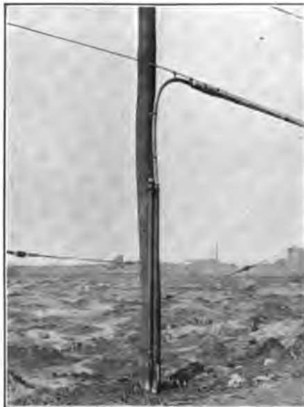
FIG. 7—CONNECTION BETWEEN AERIAL AND UNDERGROUND CABLE.
