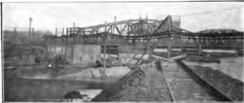
FIG. 3—AERIAL CABLE LINE WITH FIVE 13,200-VOLT CIRCUITS
