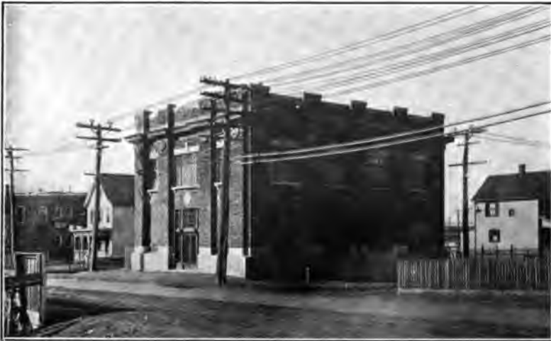
FIG. 8—AERIAL CABLE ENTRANCE TO SUBSTATION
