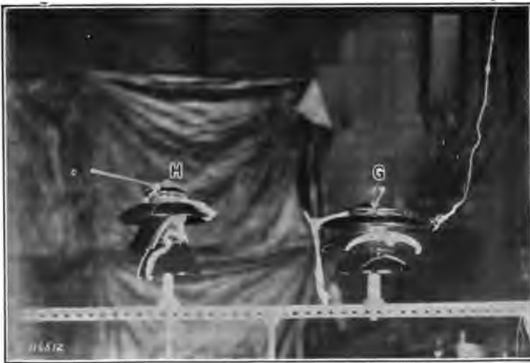
FIG. 29—SECOND SHED BROKEN—60-CYCLE DRY FLASHOVER
