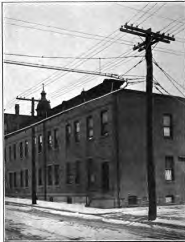
FIG. 10—CATENARY METHOD OF SUSPENDING AERIAL CABLE
