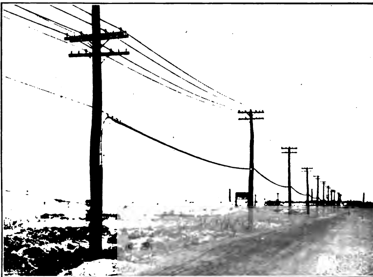
FIG. 9—28,000-VOLT AERIAL CABLE INSTALLATION [MEYER]
