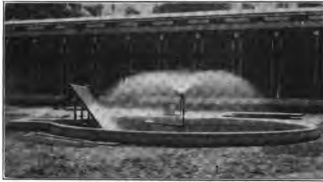
FIG. 4 THOMAS ADJUSTABLE SPRAY HEAD IN OPERATION
