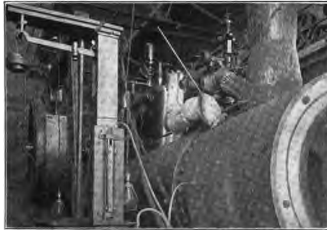
FIG. 1 TRACTION ENGINE EQUIPPED FOR TESTING, IN LABORATORY OF OHIO STATE UNIVERSITY
