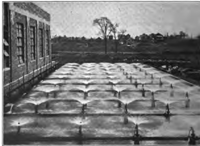
FIG 19 COOLING POND WITH ADJUSTABLE SPRAY HEADS FOR STATION OF 2500 KW. CAPACITY
