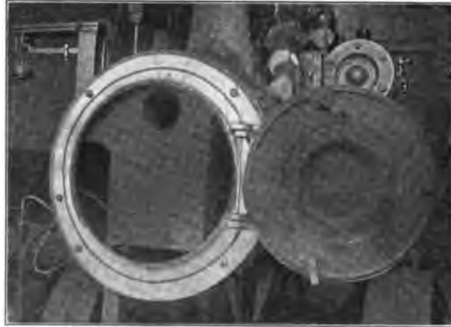
FIG. 7 SUPERHEATER IN PLACE IN SMOKEBOX OF BOILER
