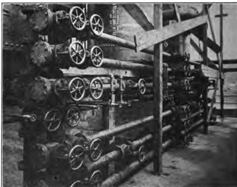
FIG. 6 OPERATING VALVES FOR DISTILLATES FROM DEPHEGMATORS
