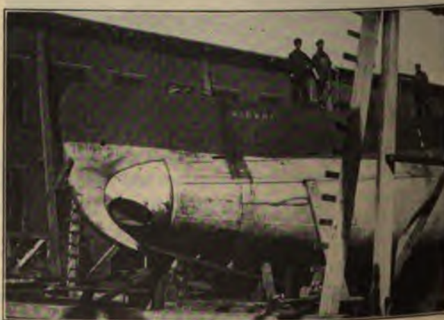
FIG. 5 BOW OF SUBMARINE WITH BOW CAP IN POSITION FOR TORPEDO FIRING
