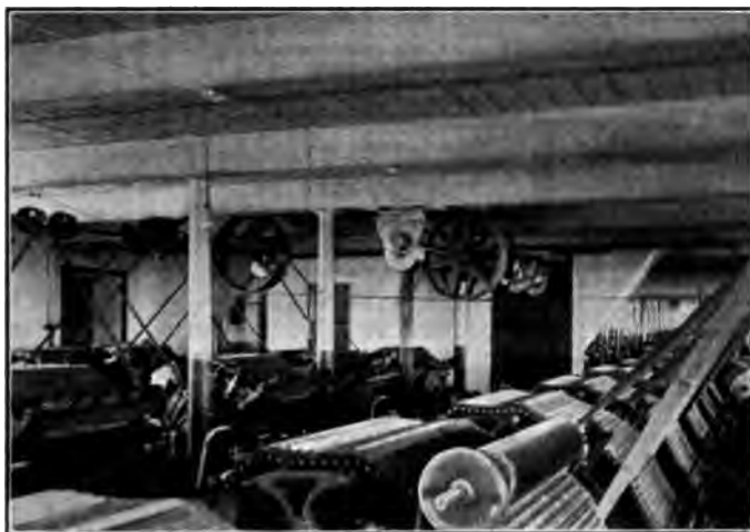
FIG. 7 CARD ROOM, THIRD STORY. ENDS SLOPED TO ECONOMIZE SPACE. NOTE WIRE GLASS WINDOW AND FIRE DOOR WITH REMOVABLE PANELS ABOVE
