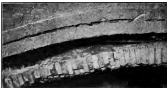
FIG. 16 VIEW SHOWING ARCH AFTER PART OF IT FELL. FALLEN PART PATCHED
