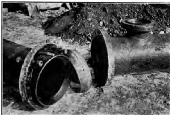
FIG. 6 VIEW OF PIPE JOINT AND WELDED NECK
