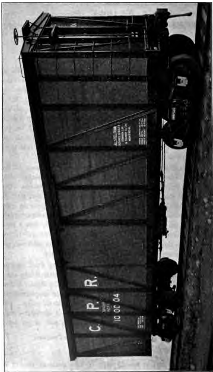
FIG. 1 FIRST INSIDE RIVETED STEEL FRAME CAR BUILT BY THE CANADIAN PACIFIC RAILWAY
