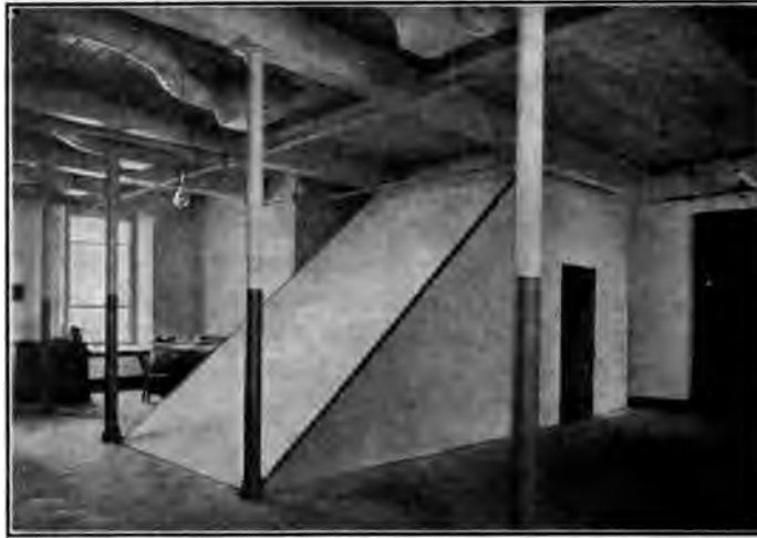
FIG. 5 HARNES ROOM, SECOND STORY, DIRECTLY OVER FLYWHEEL SHOWING PROTECTION OF BELTS LEAVING WHEEL
