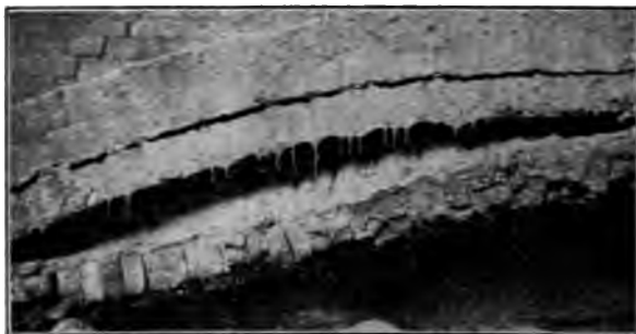
FIG. 15 VIEW OF ARCH IN SAGGED CONDITION FIVE DAYS BEFORE PART OF IT FELL
