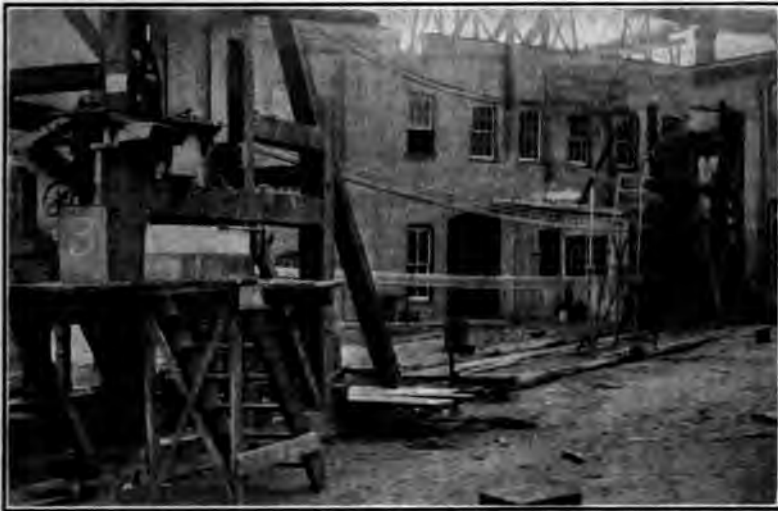
FIG. 15 AMERICAN DIFFERENTIAL DRIVE, 100 FT. ON CENTERS, SIX ROPES, 2500 FT. PER MIN., 165 H. P.
