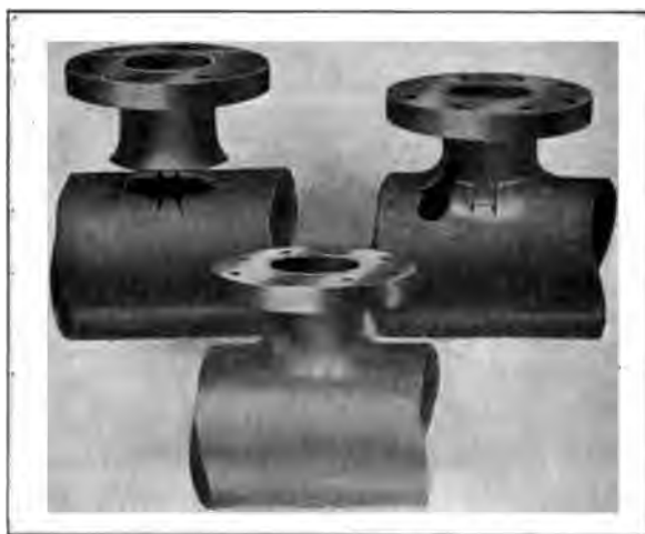
FIG. 9 DETAIL OF WELDED NECK
