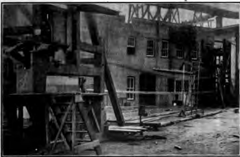
FIG. 16 AMERICAN DIFFERENTIAL DRIVE, 100 FT. ON CENTERS, SIX ROPES, 2500 FT. PER MIN., 220 H. P.
