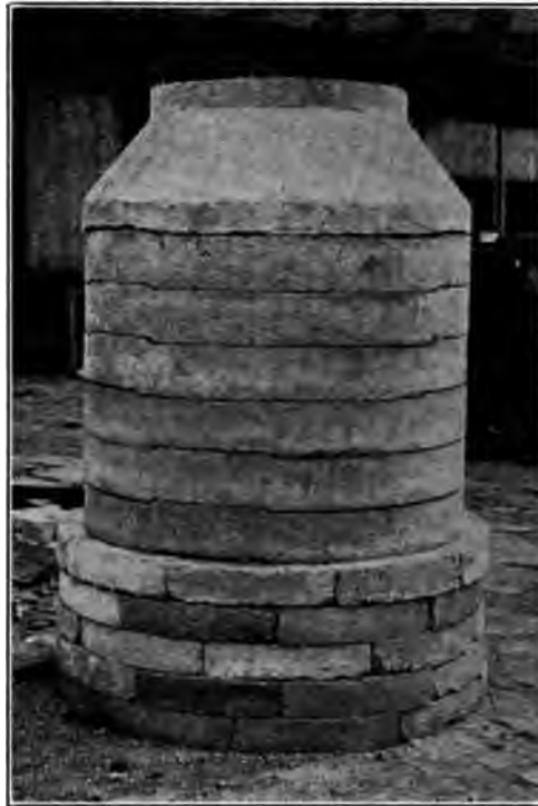
FIG. 14 CONCRETE VALVE BOX MADE UP
