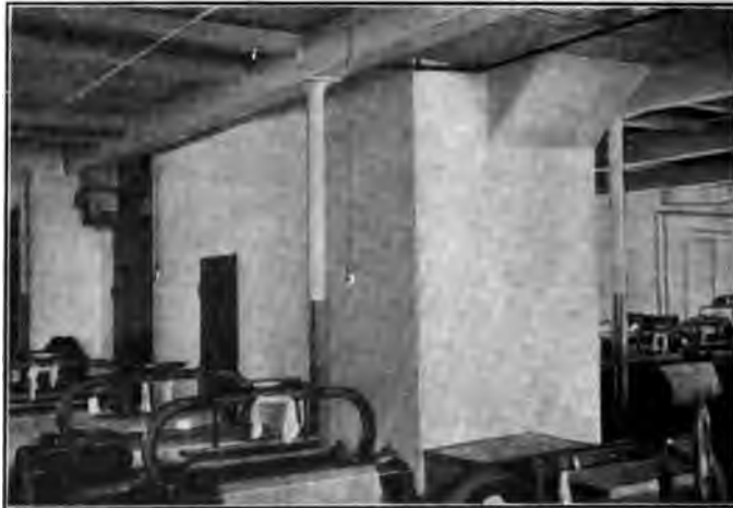
FIG. 6 WEAWE ROOM, SECOND STORY. NOTE FIRE DOOR WITH REMOVABLE PANELS ABOVE TO ALLOW ACCESS TO PULLEY ON LINESHAFT
