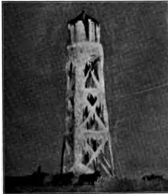
FIG. 8 UNUSUAL CASE OF LOADING OF LARGE STEEL TOWER STRUCTURE BY ICE; 60,000-GAL. TANK ON A 79-FT. TOWER, UNINJURED AFTER THAW
