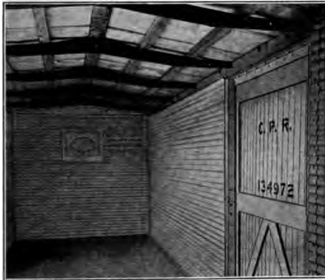
FIG. 9 INTERIOR OF CANADIAN PACIFIC STEEL FRAME CAR WITH CORRUGATED STEEL LINING
