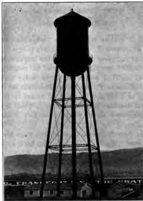
FIG. 1 TYPICAL DETACHED TOWER STRUCTURE FOR ELEVATED TANK. CAPACITY 150,000 GAL.; ELEVATION 242 FT. TO BOTTOM OF TANK
