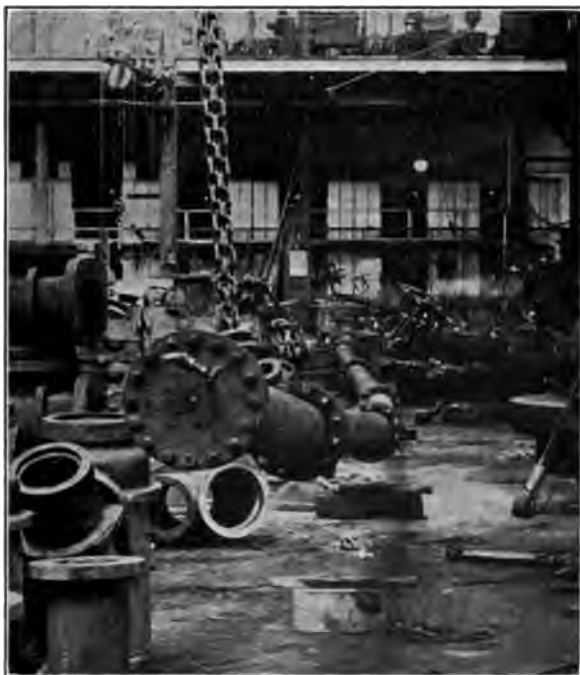
FIG. 7 SHOP TEST OF PIPE JOINT
