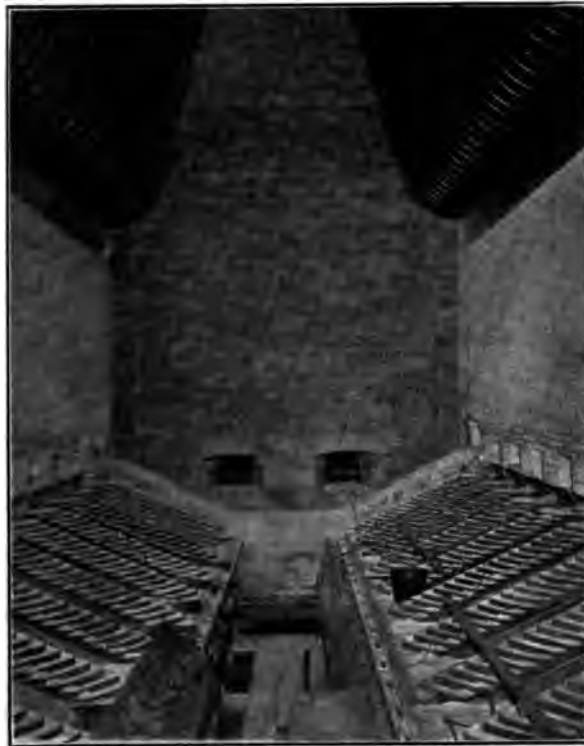
FIG. 3 INSIDE VIEW OF FURNACE WITH TAYLOR STOKER
