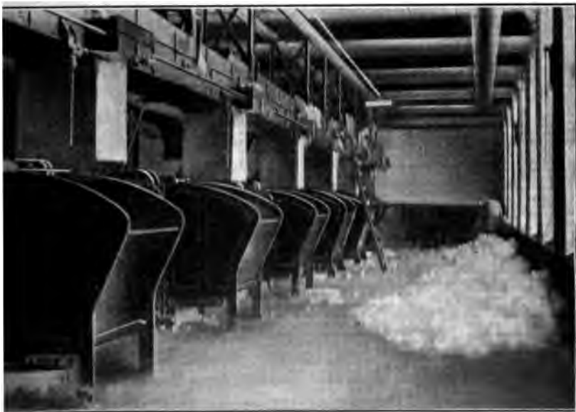
FIG. 4 PICKER ROOM WITH HOPPERS OF AUTOMATIC FEEDERS FILLED BY OVERHEAD MODERN MECHANICAL CONVEYOR
