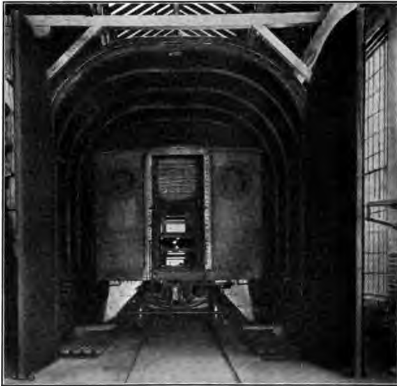
FIG. 2 VIEW OF INTERIOR OF OVEN SHOWING CAR IN PLACE
