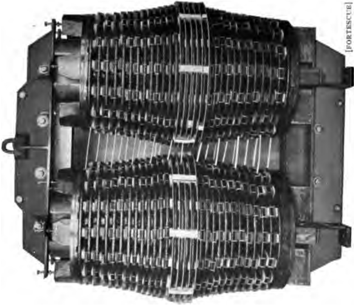
FIG. 8.—TRANSFORMER WITH EXTERNAL BARRIER REMOVED
