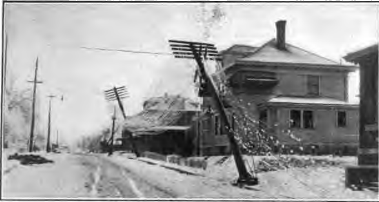
FIG. 1A—EFFECT OF SILVER THAW, PORTLAND, OREGON, 1912, ON OBSOLESCENT POLE CONSTRUCTION
