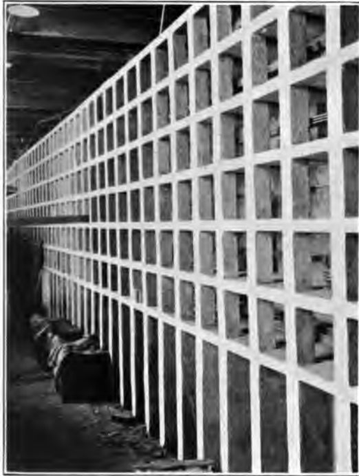
FIG. 1—SHOWING CONSTRUCTION OF GENERATOR BUS COMPARTMENTS
