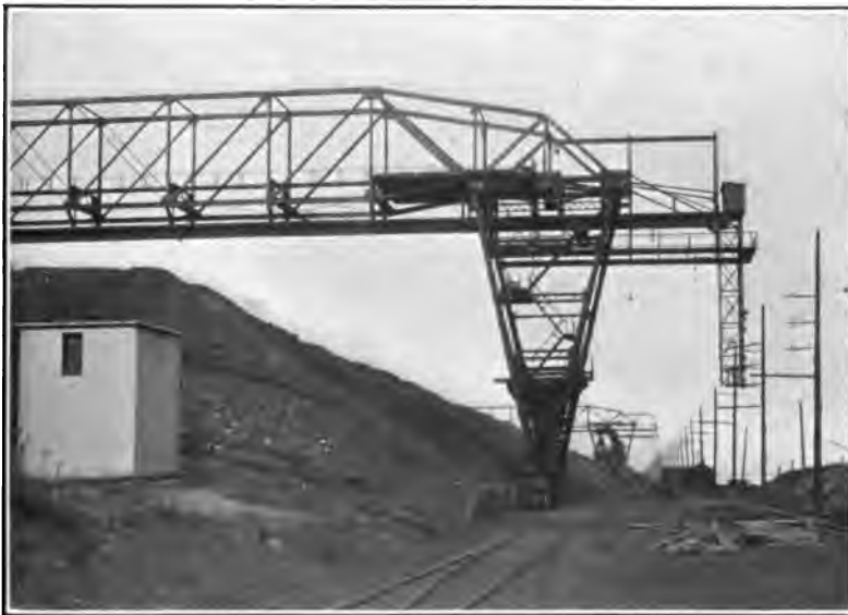
FIG. 4—MAN TROLLEY [RYERSON AND CRANE] Showing junction house, screening hopper, 13,000-volt catenary and 440-volt trolley
