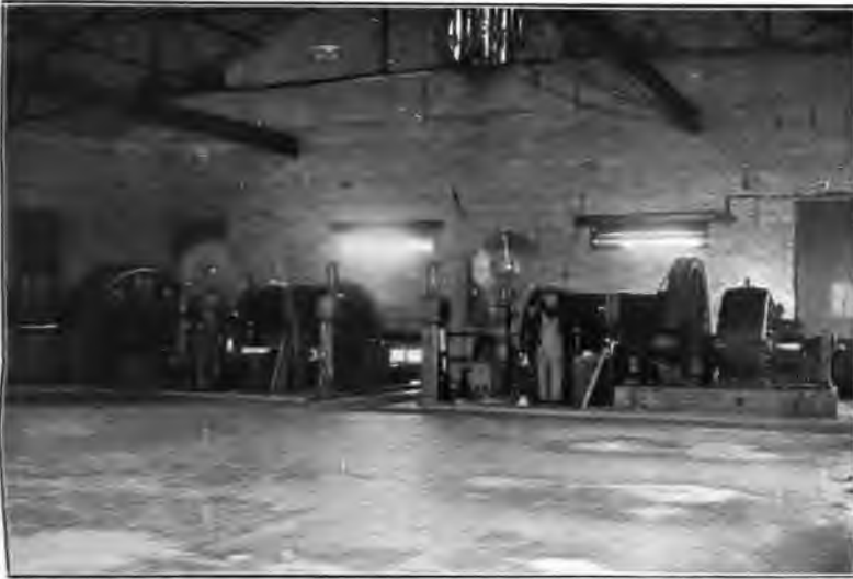
DIRECT-COUPLED ORE HOIST AND GEARED MAN AND MATERIAL HOIST Cleveland-Cliffs Iron Company, Negaunee, Mich.
