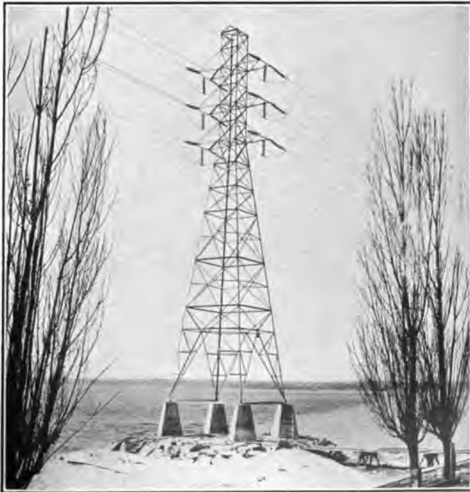
FIG. 3—INTERMEDIATE STRAIN ANCHOR TOWER. [WORCESTER] Hydro-Electric Power Commission of Ontario.
