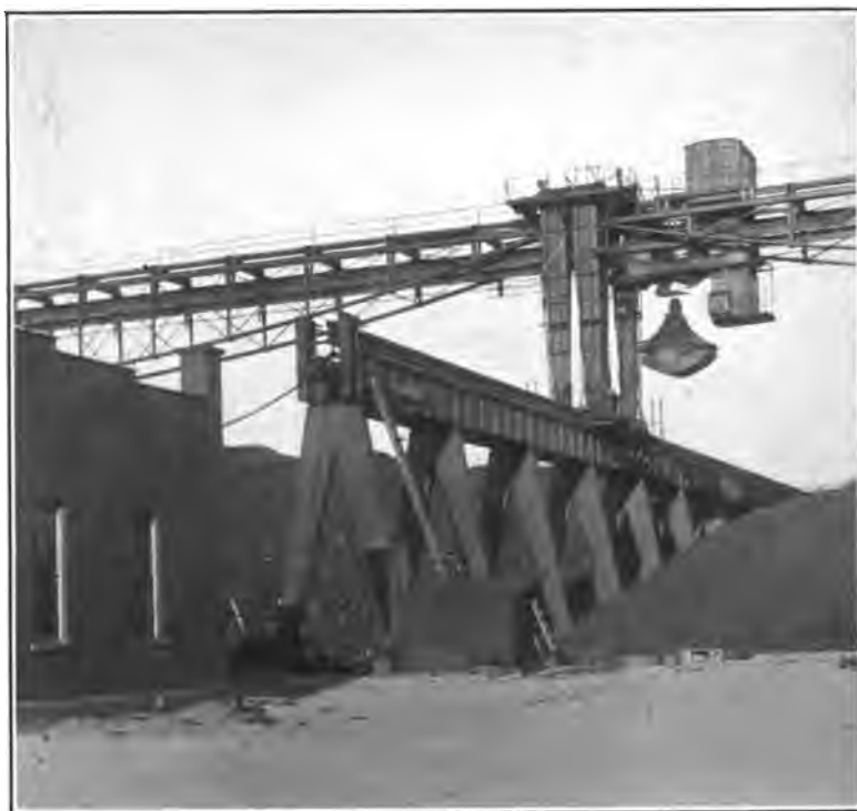
FIG. 7—MAN TROLLEY [RYERSON AND CRANE] Showing transformer house and method of distributing 440 volts to bridge
