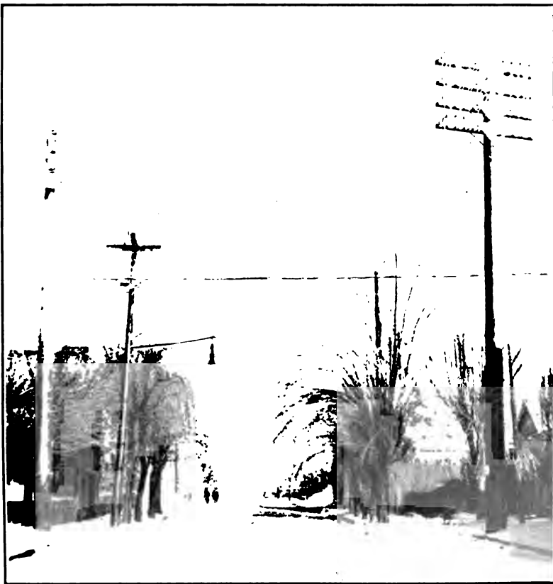
FIG. 1B—EFFECT OF SILVER THAW, PORTLAND, OREGON, 1912, ON MODERN STANDARD TOLL LINE CONSTRUCTION
