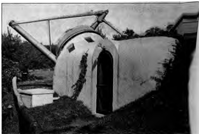
FIG. C VIEW SHOWING WEST SIDE AND SOUTH END
