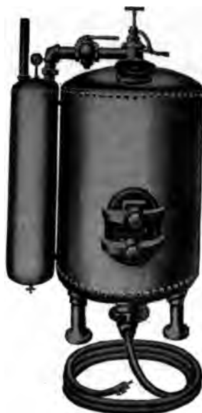
FIG. 1 SAND-BLASTING MACHINE
