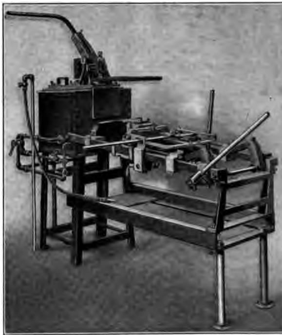
FIG. 11 SOSS DIE-CASTING MACHINE
