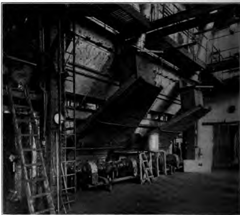
FIG. 9 SPECIAL HOPPERS AND COAL-WEIGHING SCALES
