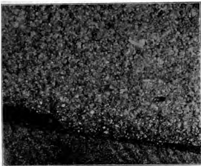
1 ROCKAWAY BEACH CORE COMPOUNDED WITH GLUTRIN SHOWING SWEATING OF THE BINDER TO THE SURFACE OF THE CORE
