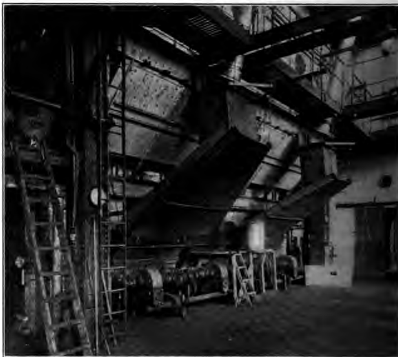
FIG. 9 SPECIAL HOPPERS AND COAL-WEIGHING SCALES
