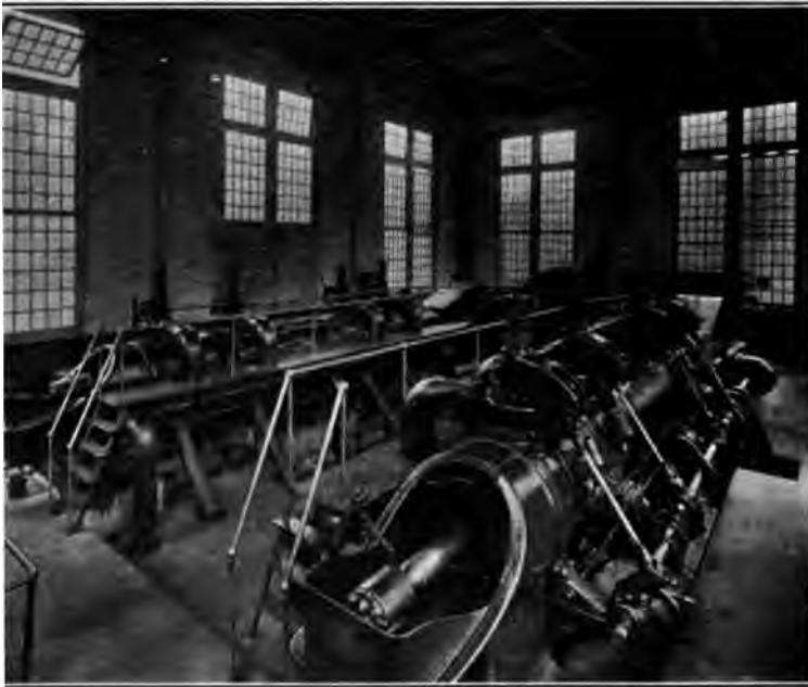
FIG. 1 INTERIOR VIEW OF THE PLANT
