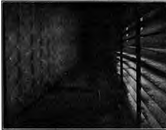
FIG. 7 HUMIDIFIER SHOWING SPRAYS IN OPERATION
