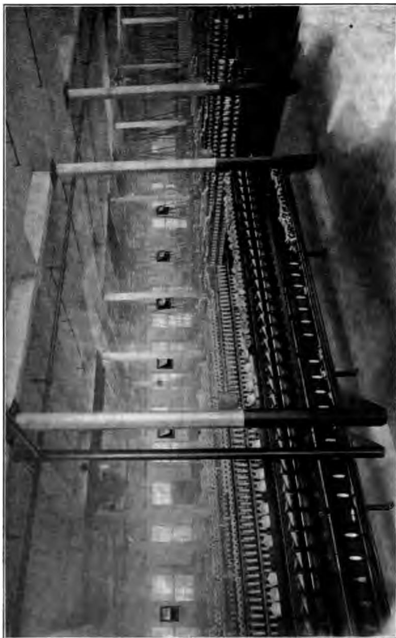
FIG 11 SPINNING ROOM SHOWING OUTLETS IN DEWPOINT AIR-CONDITIONING SYSTEMS.
