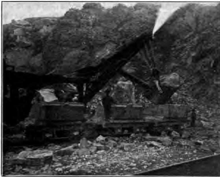
FIG. 6 STEAM SHOVEL LOADING LARGE STONES
