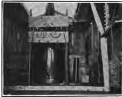
FIG. 12 (b).—Transformer end of car No. 2
