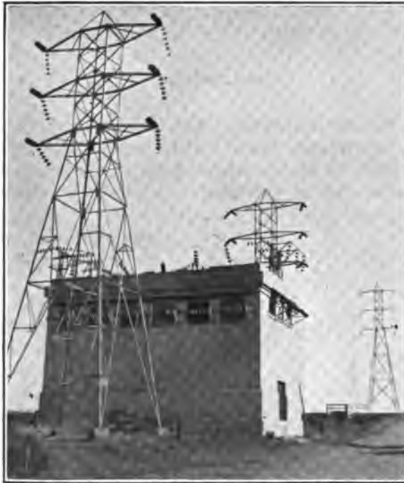
FIG. 2.—Transmission line of Great Western Pr. Co. at Brighton
