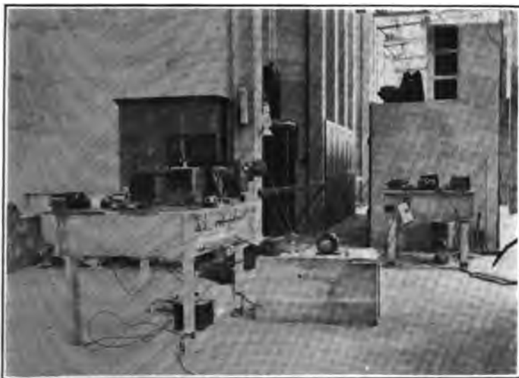
FIG. 18.—Oscillograph and testing equipment at Big Bend
