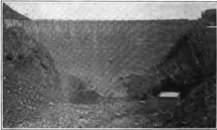
FIG. 21.—Roosevelt dam showing power house and transformer house in foreground.
