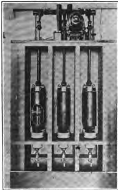
FIG. 7.—Modern high capacity, moderate voltage oil circuit breaker
