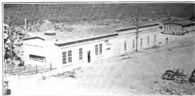
FIG. 10.—Pumping station No. 2, Minidoka project.
