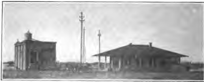
FIG. 29.—Substation, pumping plant and operators house.
