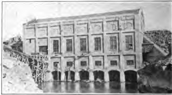
FIG. 4.—Exterior, Minidoka power house.
