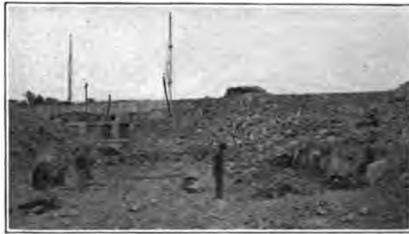
FIG. 6.—Tail race excavation, Minidoka power house.
