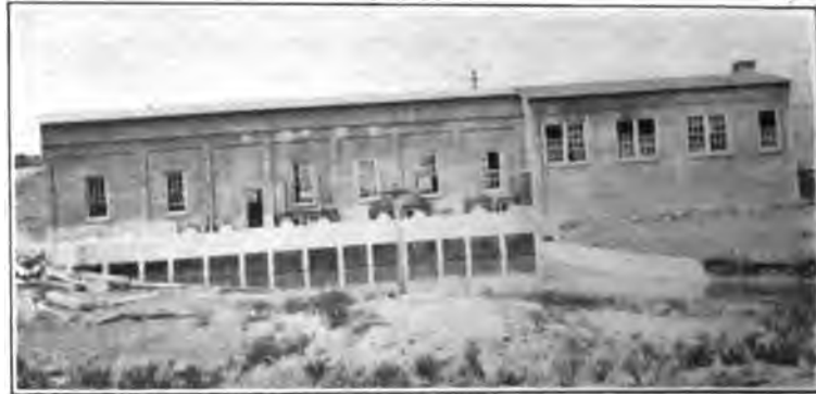
FIG. 9.—Pumping station No. 1, Minidoka project.
