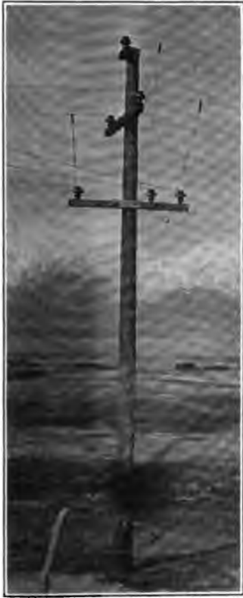
Method of connecting portable substation to 33,000-volt transmission line
