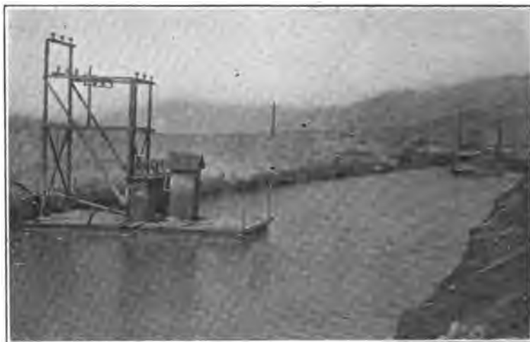
Floating transformer station used in connection with suction dredge; Owens Valley
