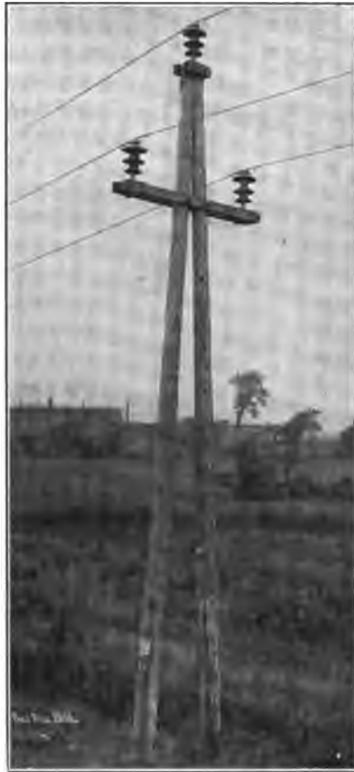
FIG. 4.—35-ft. wooden A-frame structure
