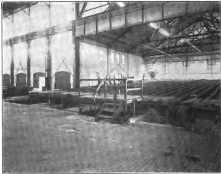
FIG. 15—Hot bed with pulpit containing master switches for rake-offs and drag-outs
