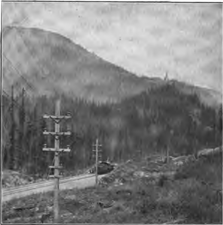
FIG. 7.—General view of transmission line
