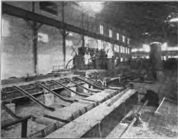
FIG. 11—Three-high blooming mill with motor-operated elevating table
