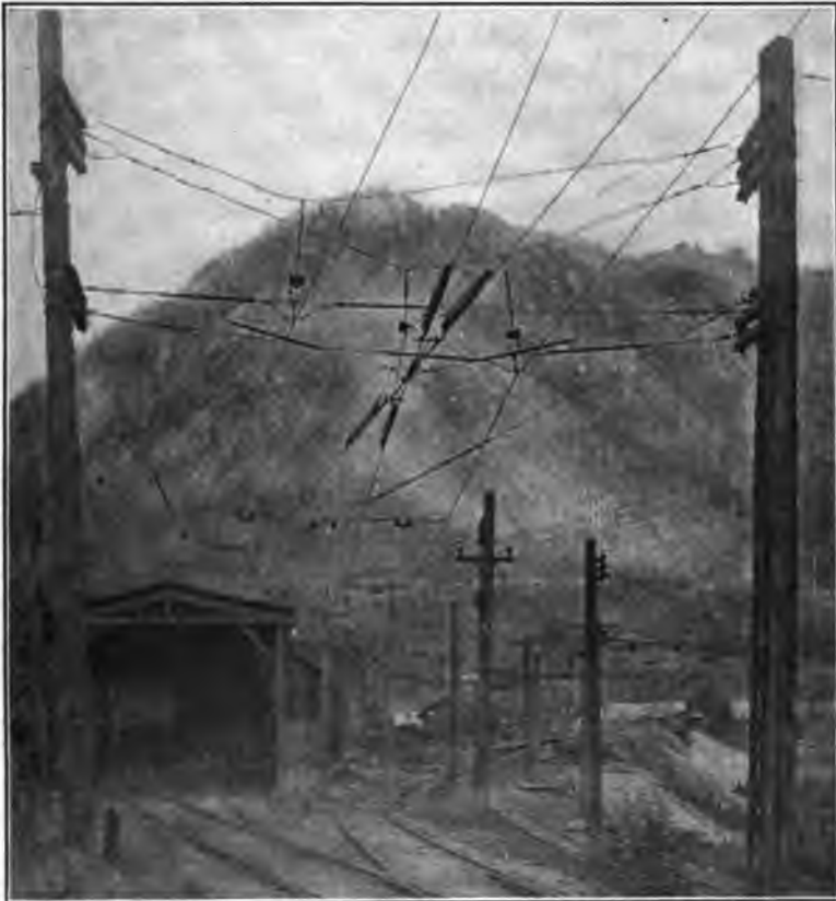
FIG. 15.—Construction at switch point, Wellington yard
