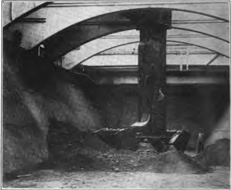
FIG. 3—Bucket leg of an ore unloader working in the hold of a steamer
