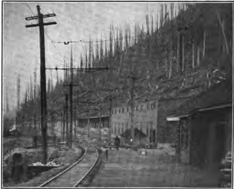
FIG. 16.—Bracket construction at curve Wellington yard
