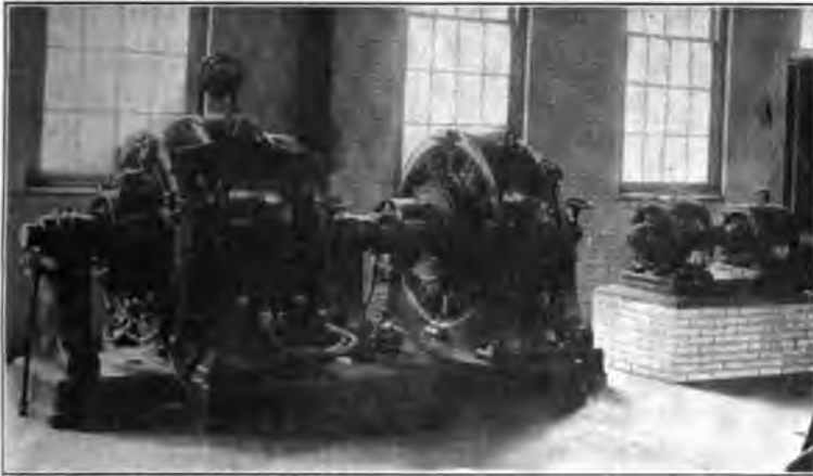
FIG. 6.—Booster and exciter, Indiana Steel Co., Gary, Ind.
