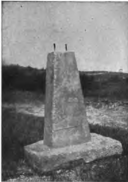
FIG. 18—Tower foundation dug up for purpose of relocation
