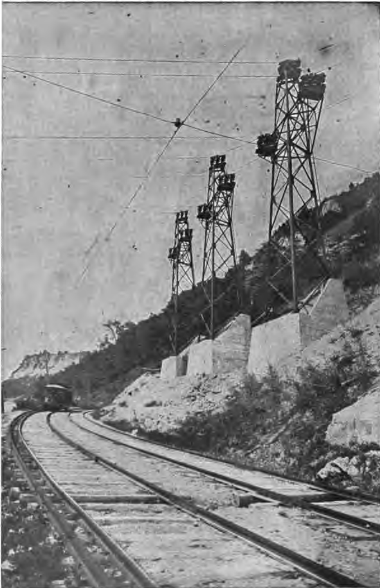
FIG. 2—Niagara crossing, water-edge towers, American side
