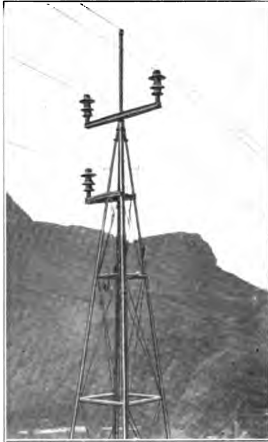
FIG. 3—Showing present appearance of line. Lightning-rods removed.
