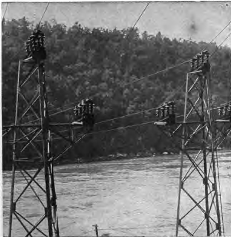
FIG. 3—Niagara crossing top of water edge towers
