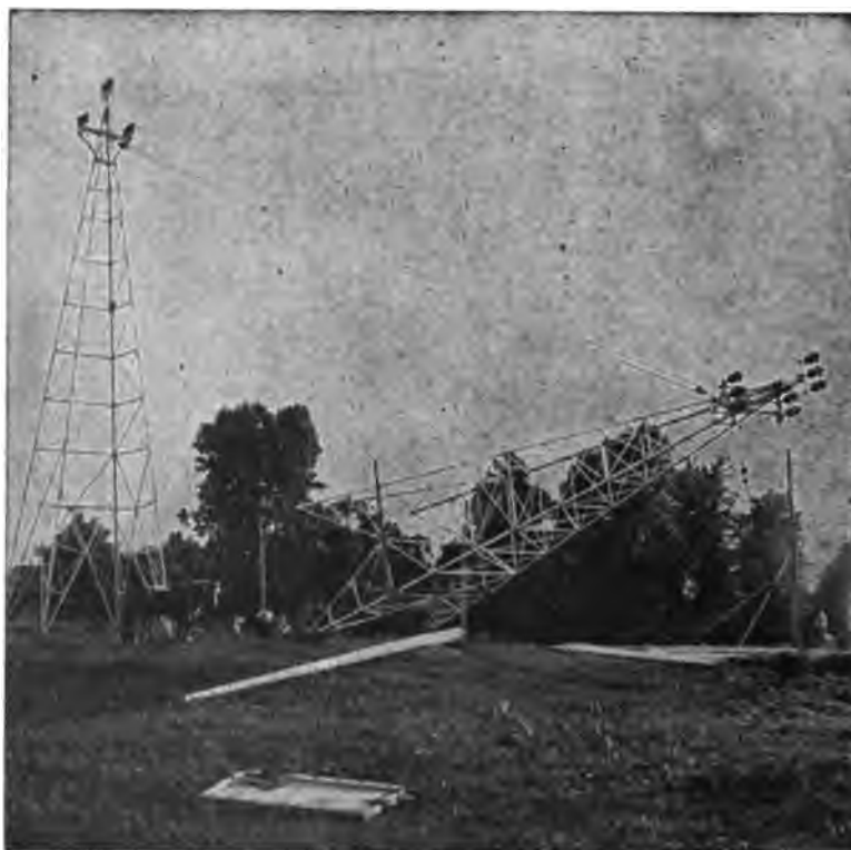
FIG. 20—Erecting 75-foot tower (2)
