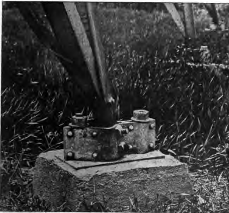
FIG. 17—Foot of tower, showing method of fastening tower to foundation
