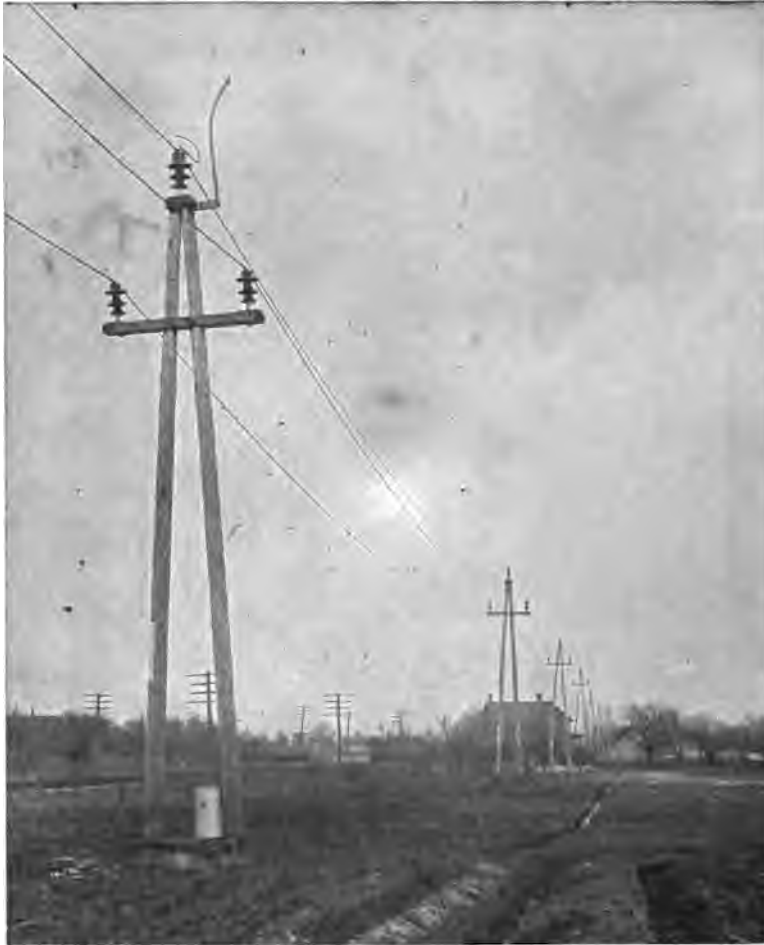
FIG 26—Standard A-frame construction showing line structure lightning-arrester
