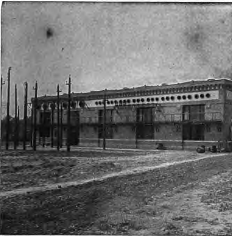
FIG. 31—Lockport sub-station showing 11,000-volt outdoor lightning-arresters
