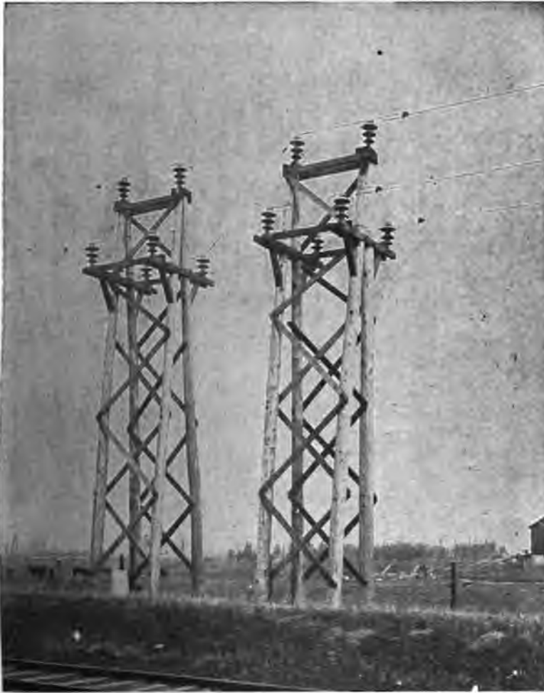
FIG. 29—A-frame transposition
