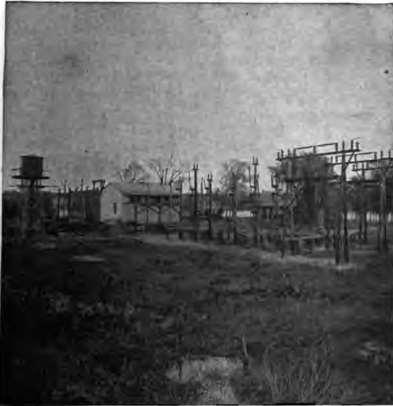
FIG. 37—Baldwinsville sub-station, showing lightning-arresters
