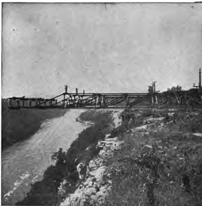
FIG. 4—Niagara crossing, cantilevers, American side
