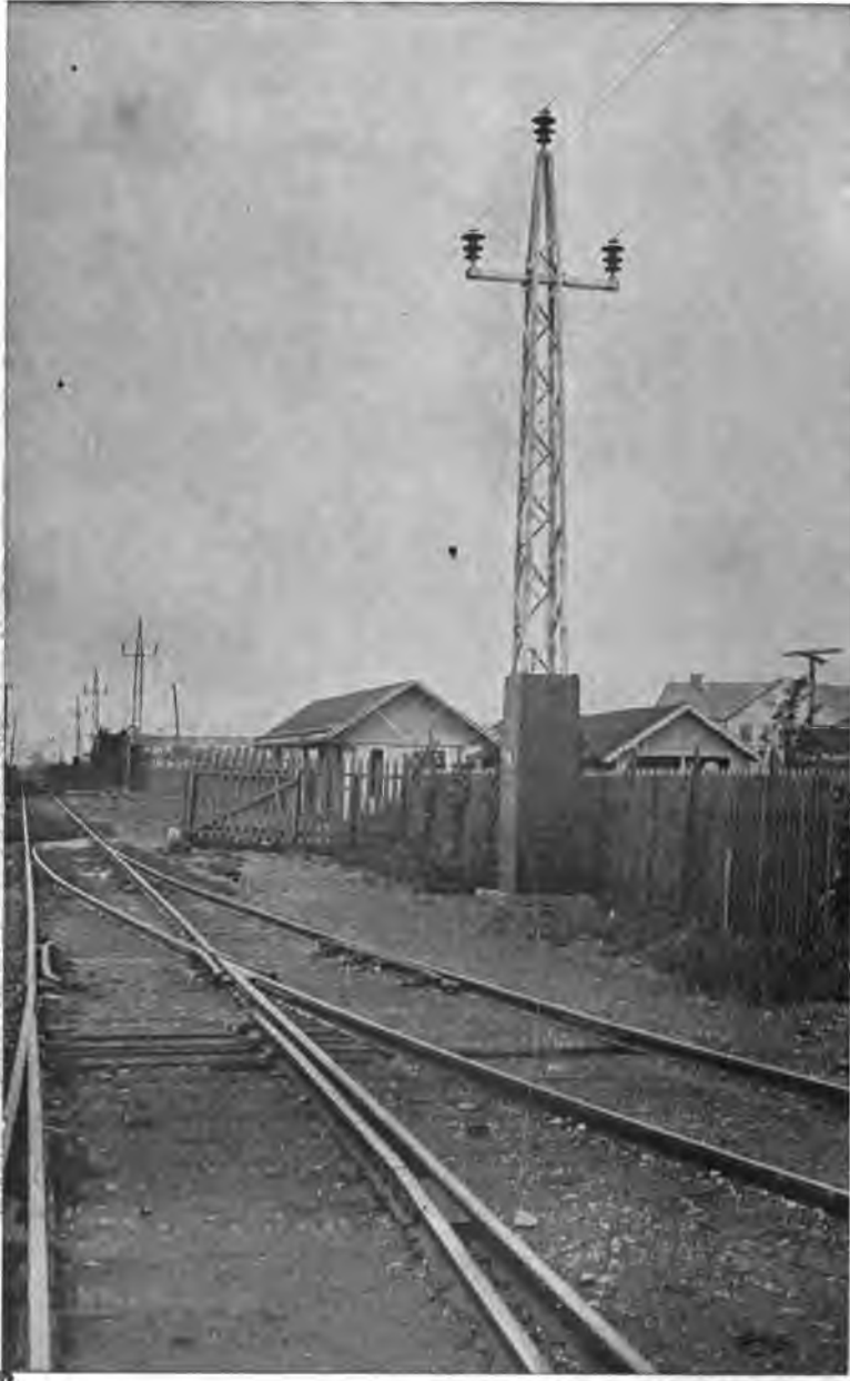
FIG. 30—Galvanized steel poles on railway
