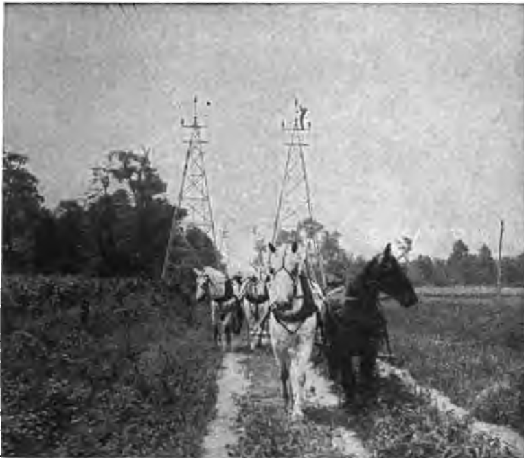
FIG. 13—Stringing line cable
