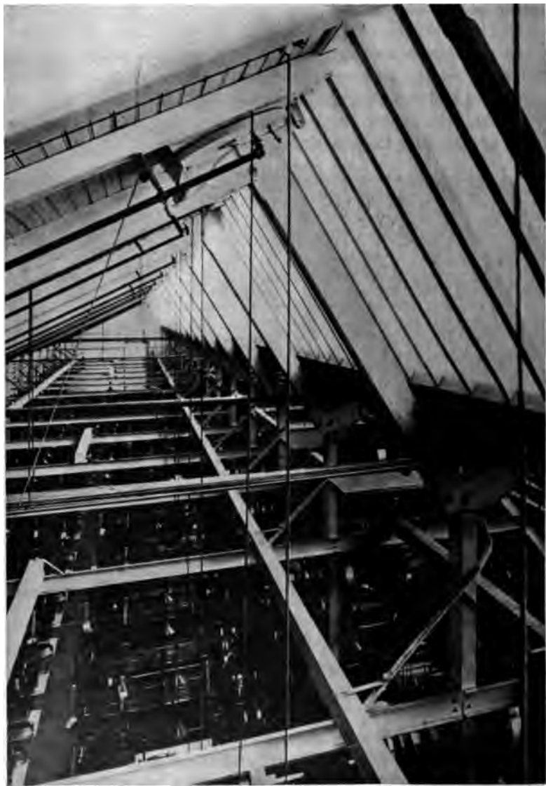
FIG. 4 INTERIOR VIEW OF SAW-TOOTH SKYLIGHT SHOWING CONSTRUCTION OF VENTILATOR DAMPERS
