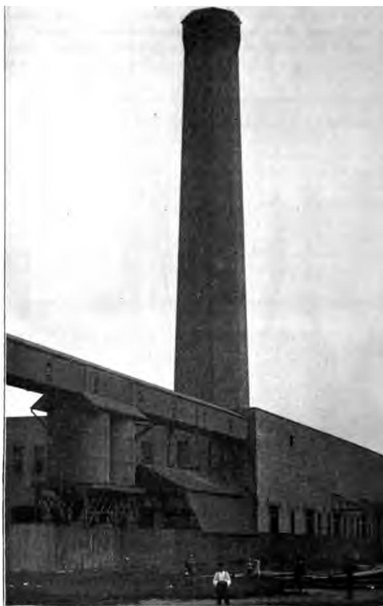
FIG 6 PLANT OF NORTHWESTERN ELEVATED RAILROAD COMPANY, OF CHICAGO. WATER TURBINES, BOILERS AND MURPHY FURNACES
