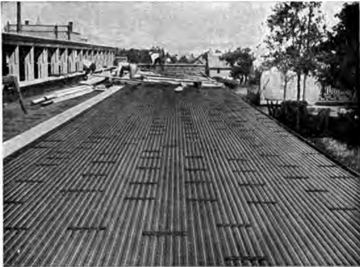
FIG. 5 ROOFS WITH FERROINCLAVE IN PLACE READY FOR CEMENTING
