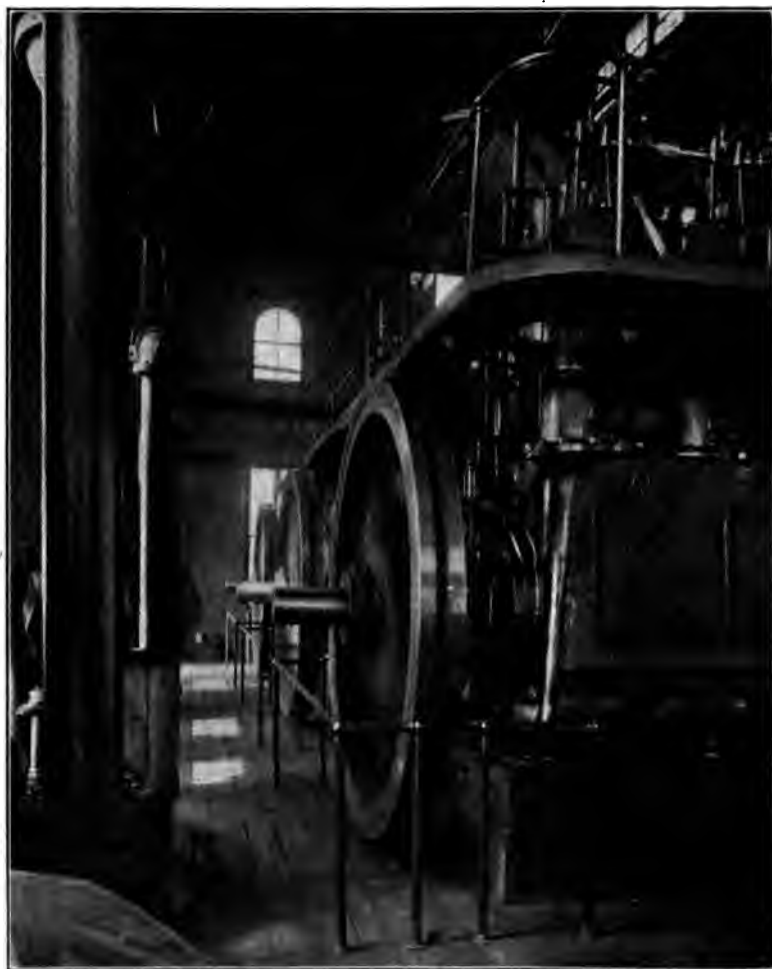
FIG. 8 ENGINE ROOM SHOWING GAS PIPING AND POSITION GAS REGULATORS
