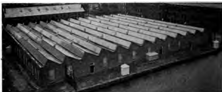
FIG. 2 EXTERIOR OF TEXTILE MILL, SHOWING SAW-TOOTH SKYLIGHT ROOF CONSTRUCTION
