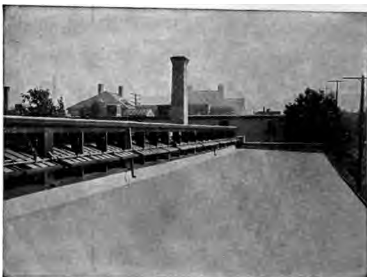
FIG. 6 ROOF CEMENTED FOR WATERPROOF COVERING
