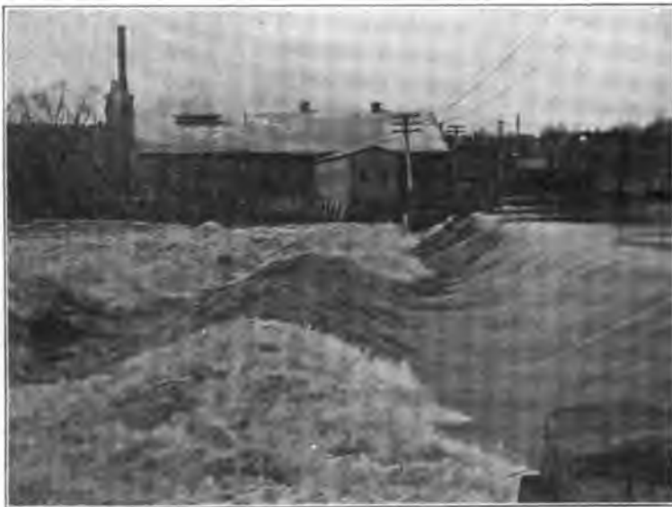
FIG. 3.—Upper dam and Central plant.
