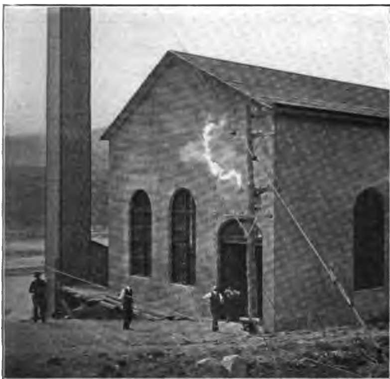
FIG. 5. Telephone Protective Device Test; 6 ft. 25-Ampere Fuse.
