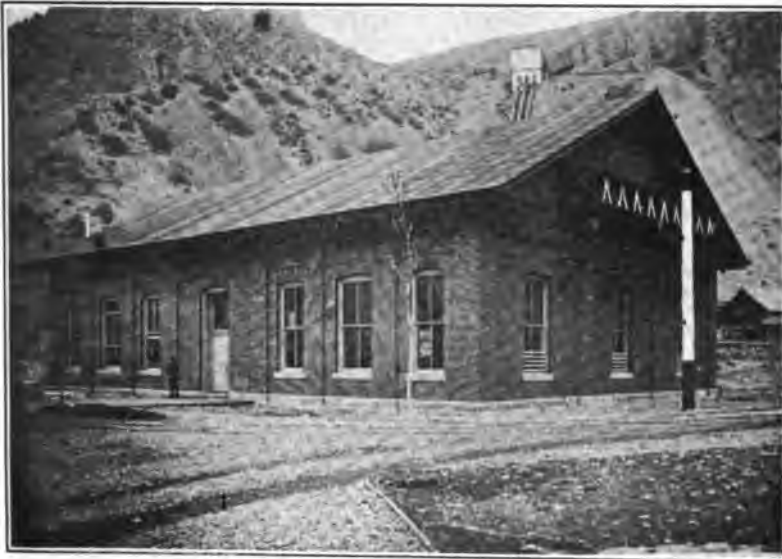
FIG. 5.—Power House at Olmsted, Utah. 10,000 h.p. capacity; line pressure 44,000 volts.
