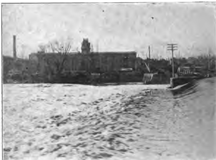
FIG. 2.—Upper dam and site of present Central plant, during progress of concrete work.
