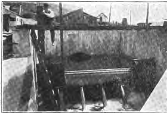
FIG. 9.—Main weir with hook gauge measuring apparatus.
