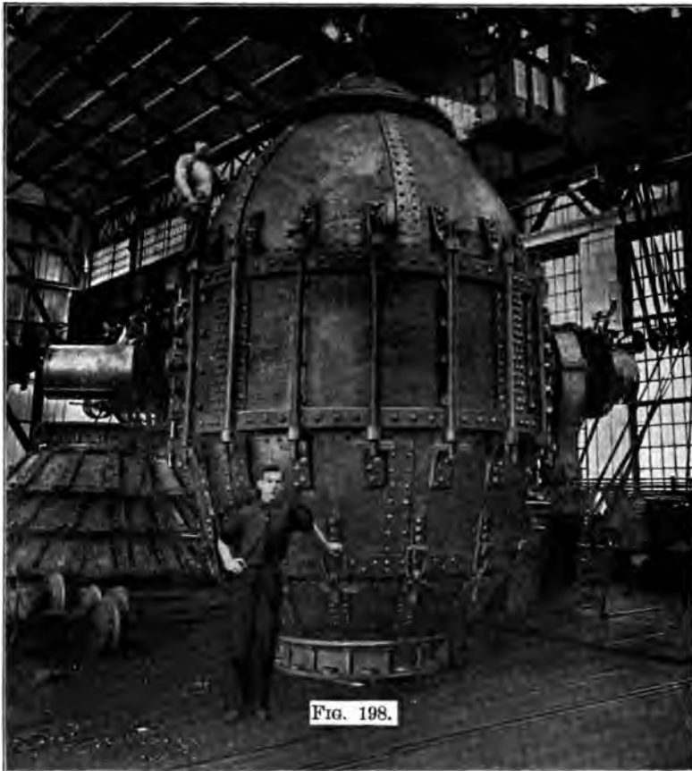
Prof. F. R. Hutton. —Fig. 198 shows the elevation of an eighteen-ton converter used at the Maryland Steel Works at Sparrow's
