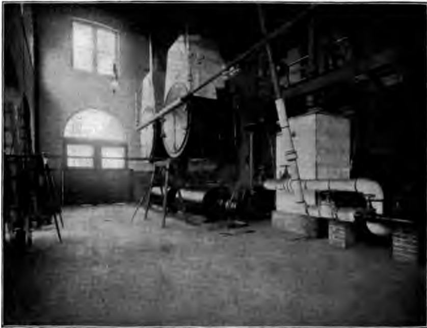
FIG. 178.—78-INCH FIRE-TUBE BOILER, POPE TUBE WORKS.
