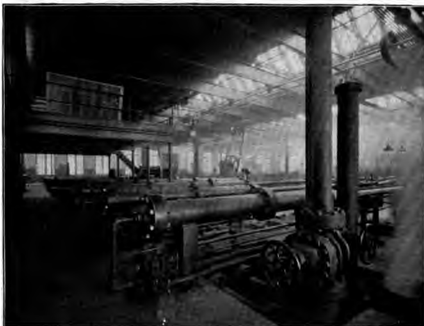
FIG. 165.—HYDRAULIC DRAW BENCHES, POPE TUBE CO.
