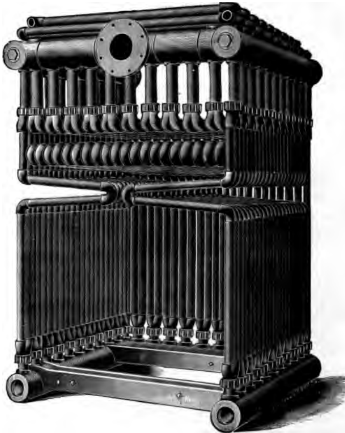
FIG. 297.—ALMY WATER TUBE BOILER, CLASS D.
