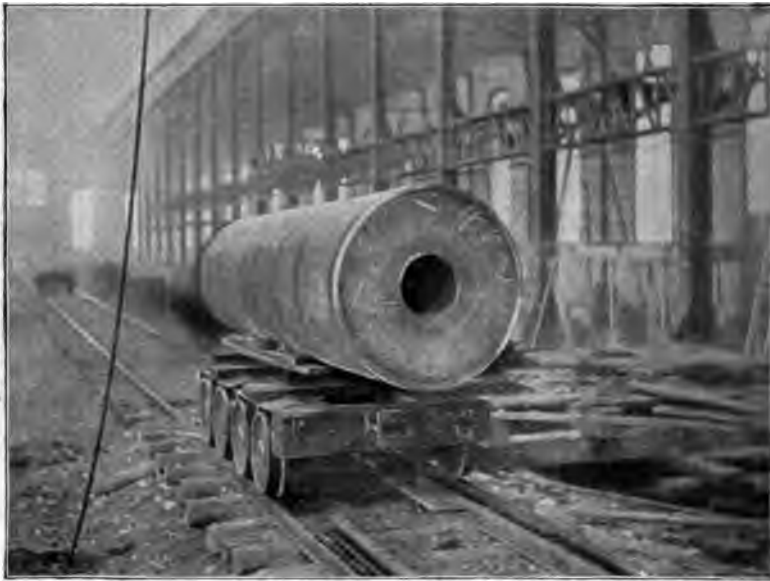
FIG. 68.—Bored ingot.
