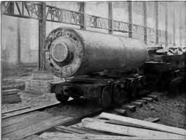
FIG. 65.—Ingot solid as coming from the mould.
