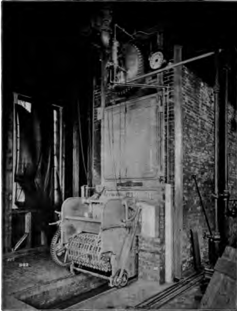
FIG. 125.—FRONT OF CHAIN-GRATE STOKER, BABCOCK & WILCOX PATTERN.
