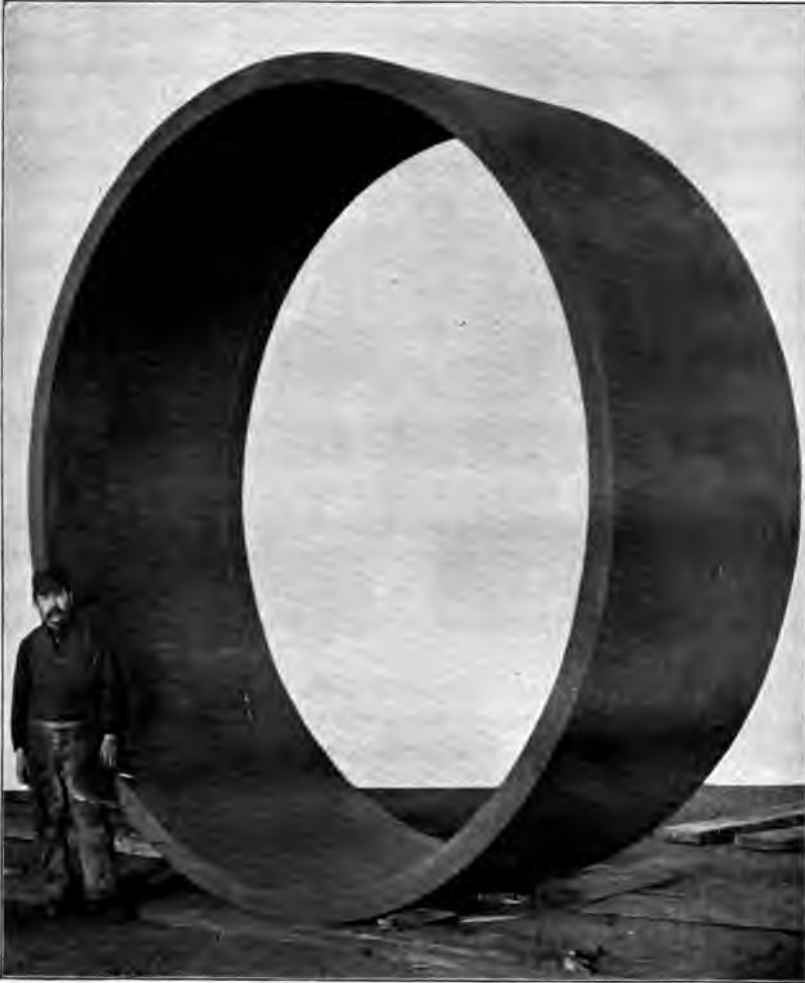
FIG. 73.—Field ring for 5,000 horse-power dynamo.
