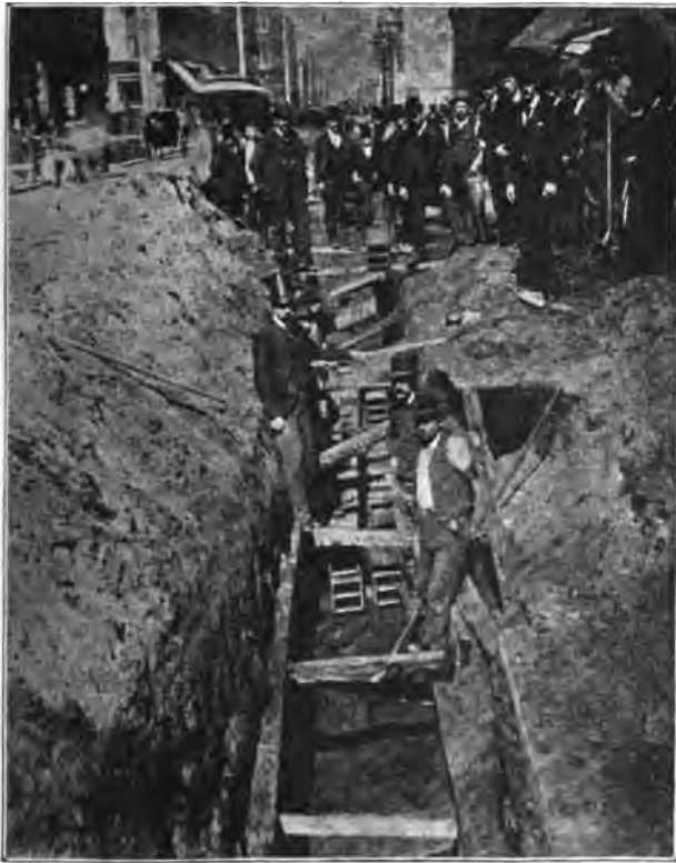
Fig. 95. Laying 10" \times 10" Ducts.
