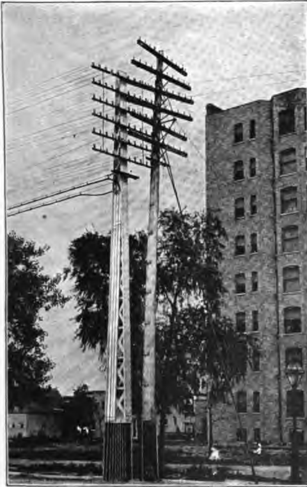
Fig. 13. Structural Iron Anchor Pole.
