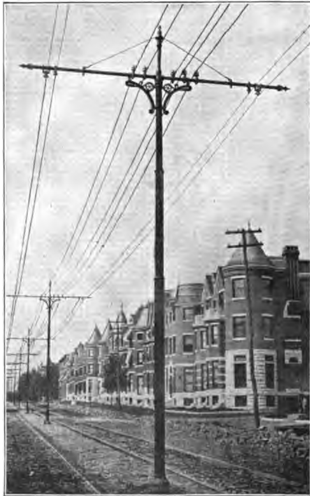
Fig. 38. Center Pole Construction.
