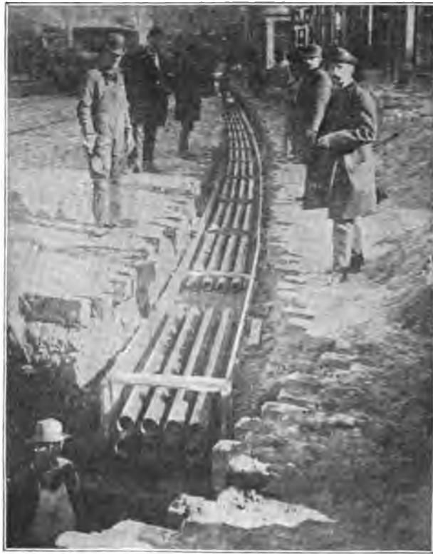
Fig. 92. Cement-lined Iron Pipe.
