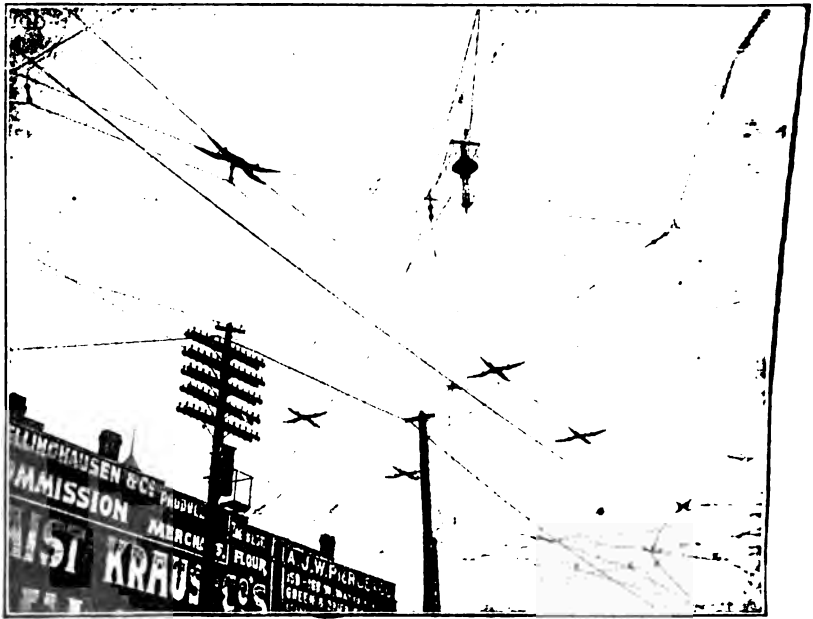
Fig. 79. Cross-overs and Switches in Place.
